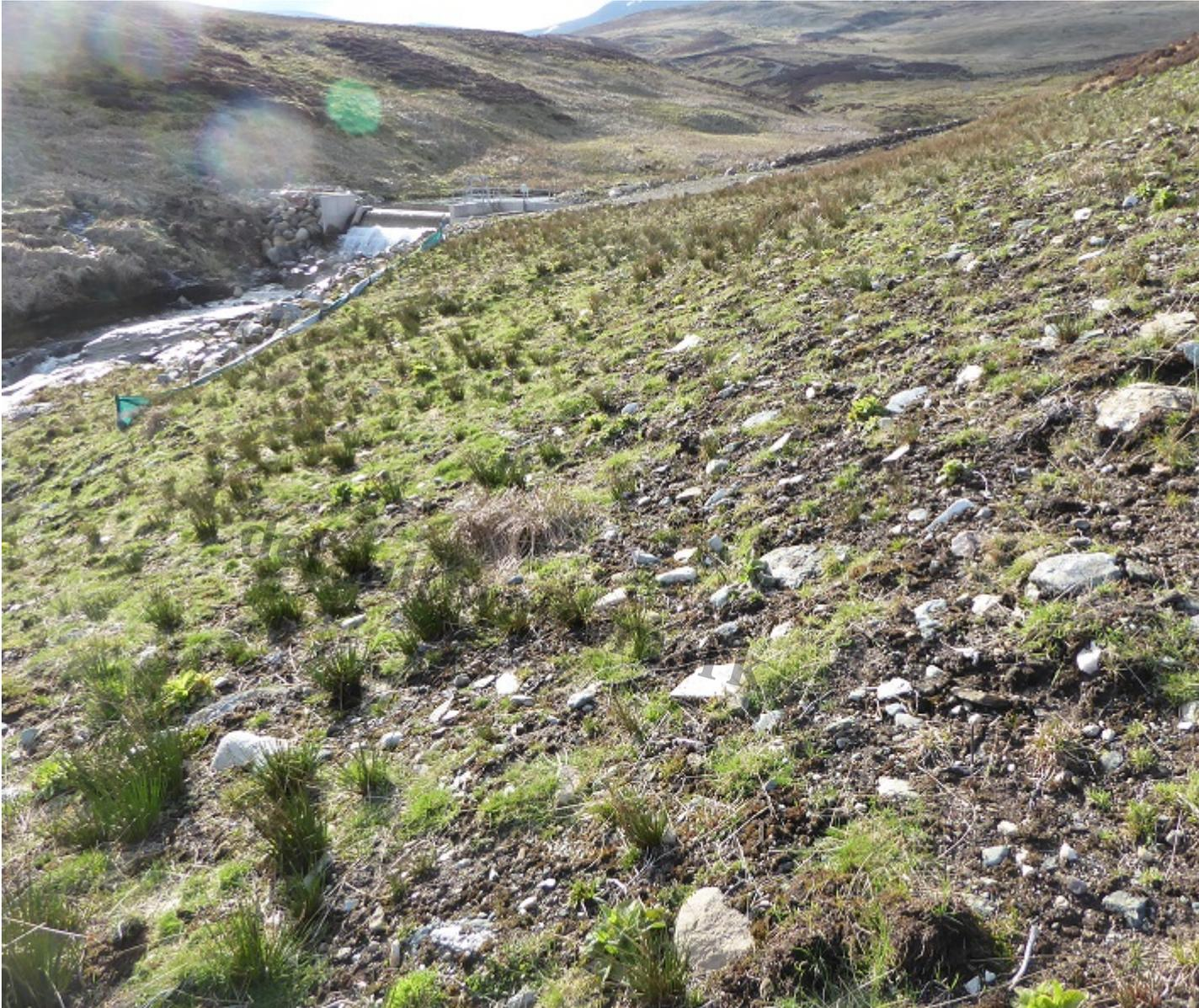
Tulchan Estate hydro showing area above the pipeline which appears to have been destroyed â?? in planning application it had stated the width of disturbed ground would be 4 metres; its over 10 metres
