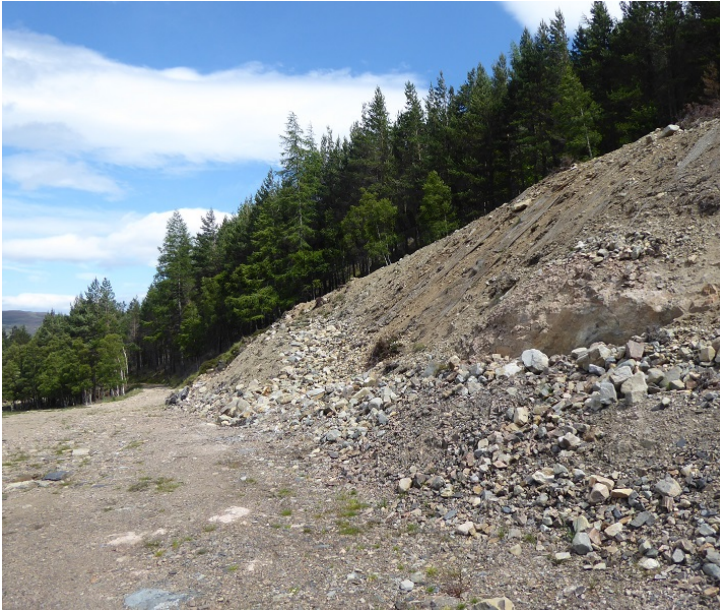
The slope by the main Corriemulzie intake in July 2017 – note how the geotextile, centre, has failed the slope and the wide area for vehicle use below
