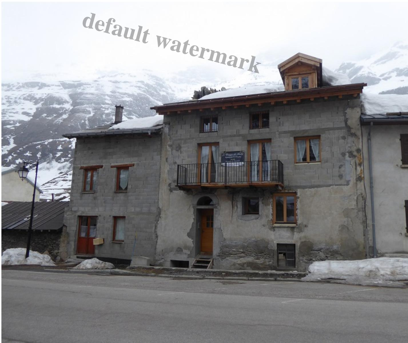
Unfinished building renovation/extension Bessans – note how concrete masonry blocks have been used to extend far older walls
