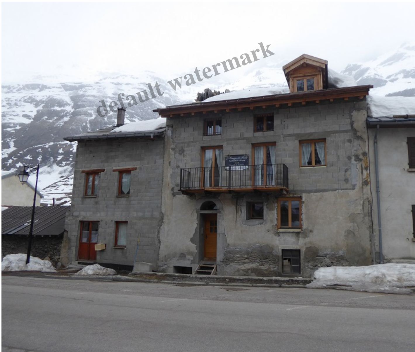
Unfinished building renovation/extension Bessans – note how concrete masonry blocks have been a
