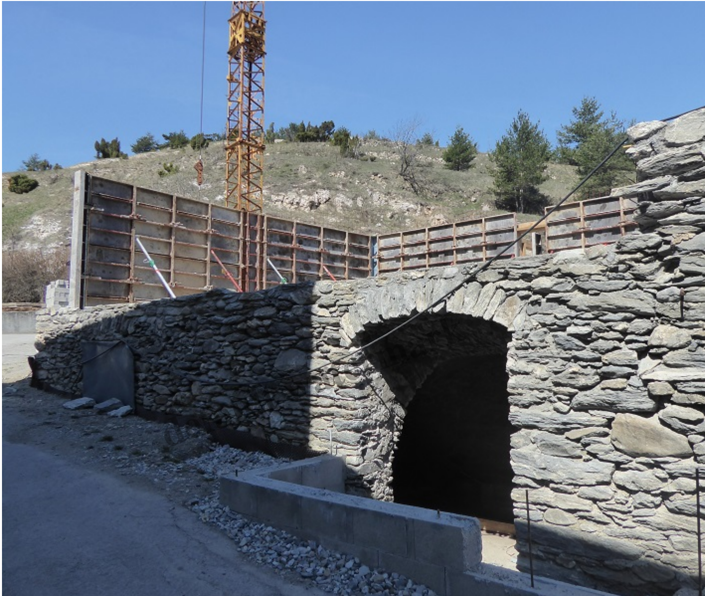
Old “cave” at Bramans which has been renovated to provide base to new building.
