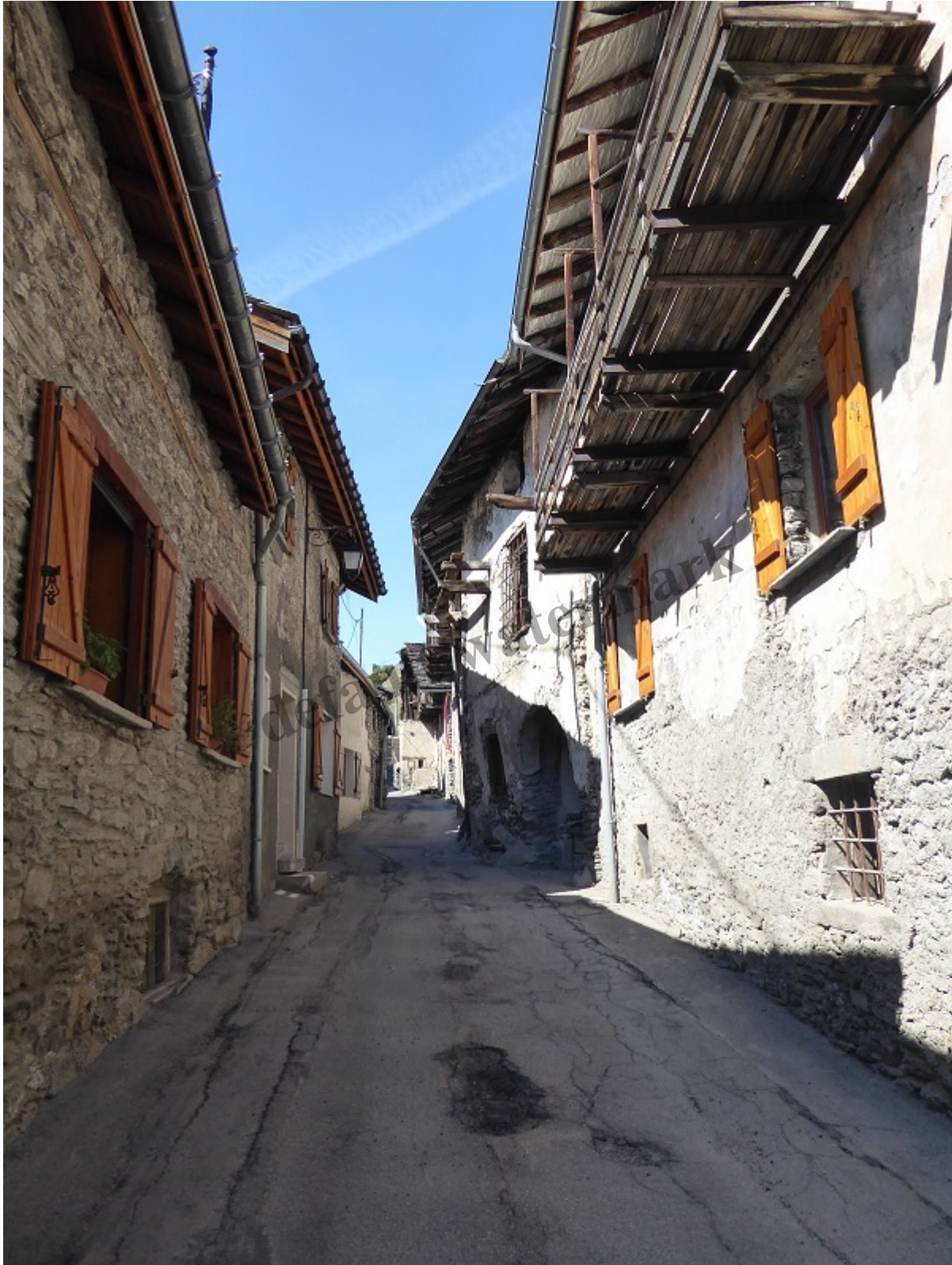
One of the main streets in Bramans where traditional houses have been renovated
