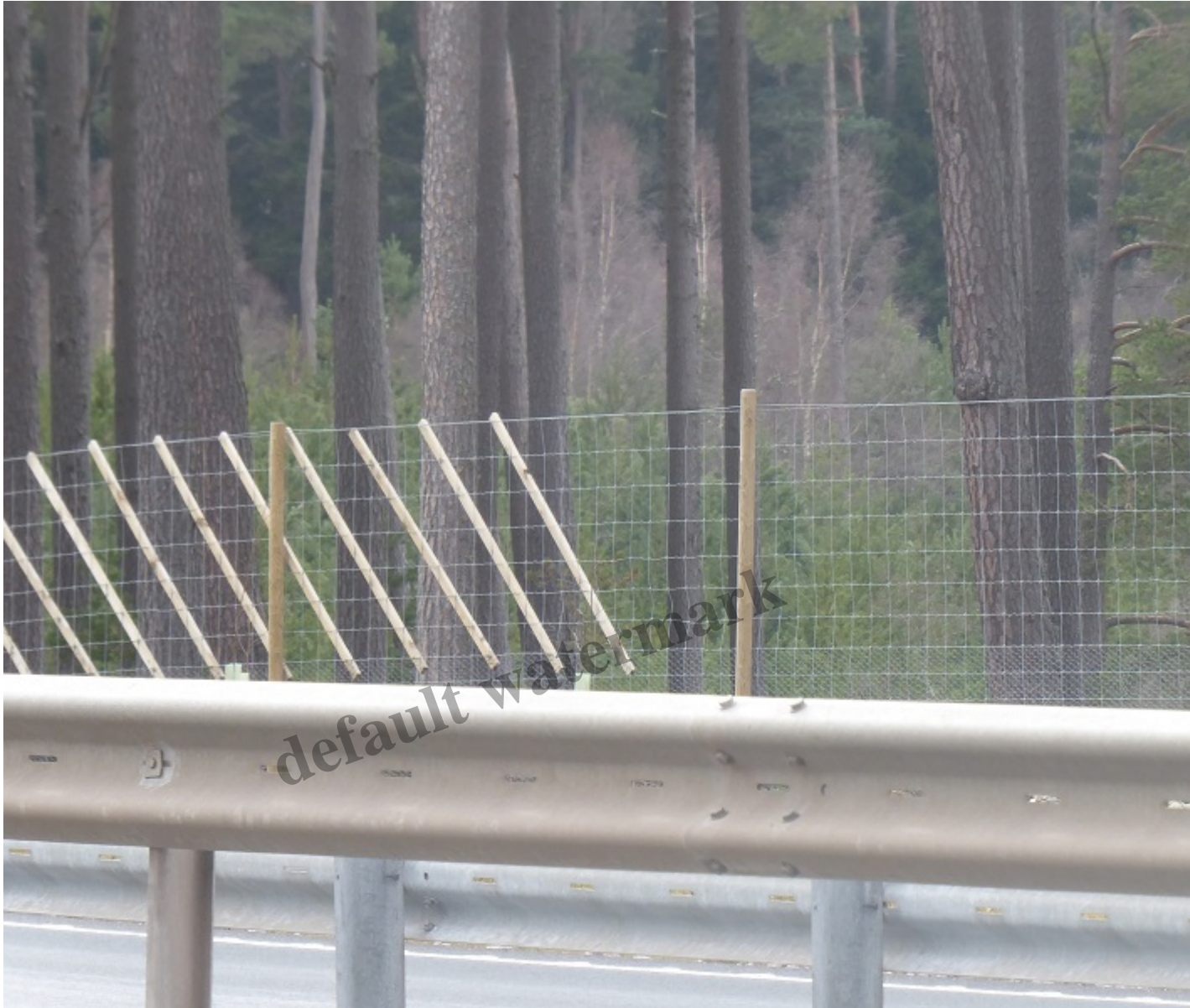
Boundary between marked and unmarked deer fence opposite south bound layby
