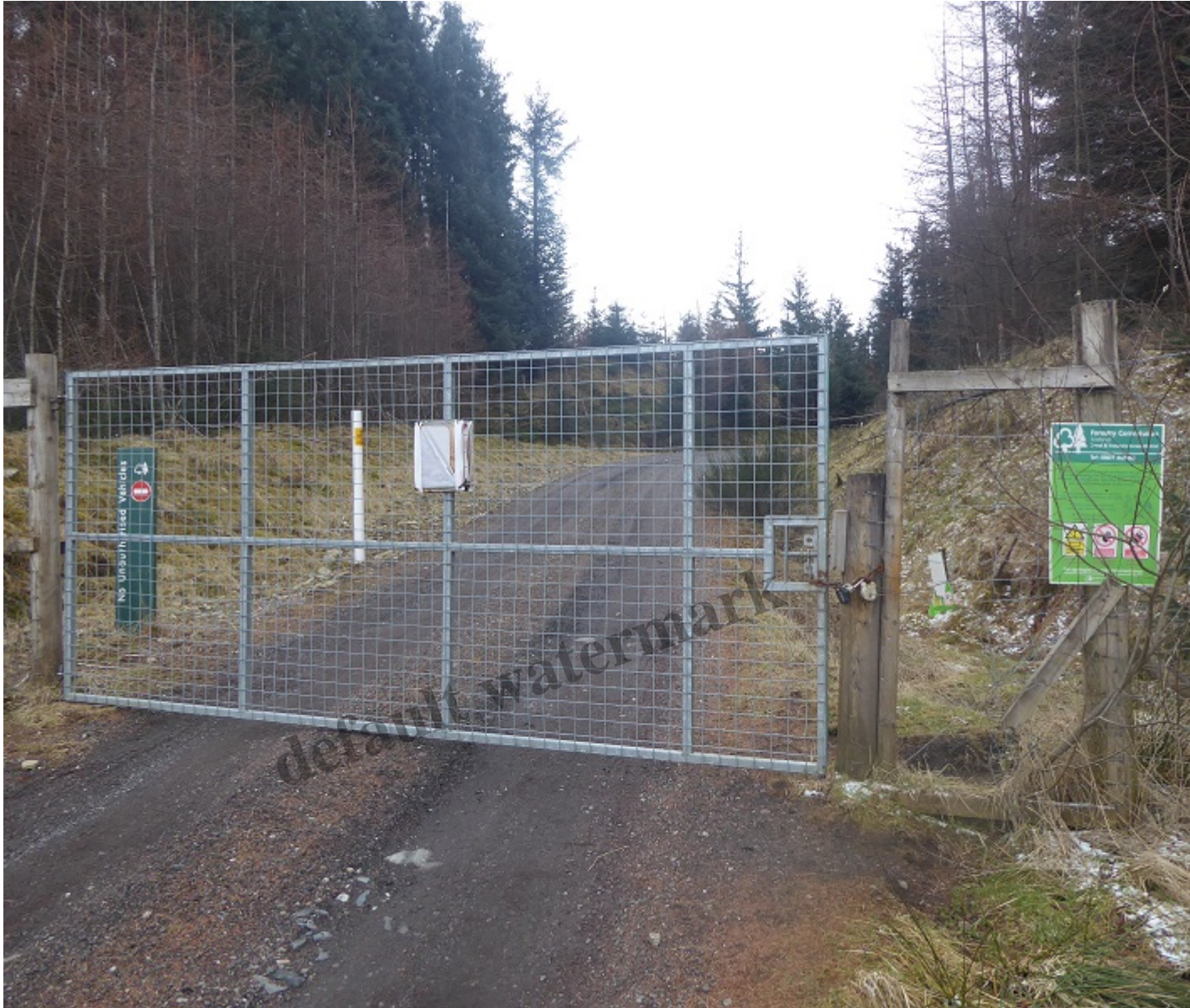
Note the padlock and lack of any means to cross/pass through the fence
