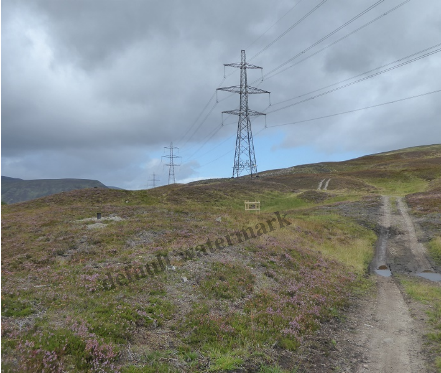
The southern end of the Dalnacardoch track above Dalnaspidal before the section which has been “ which starts by the first tower
