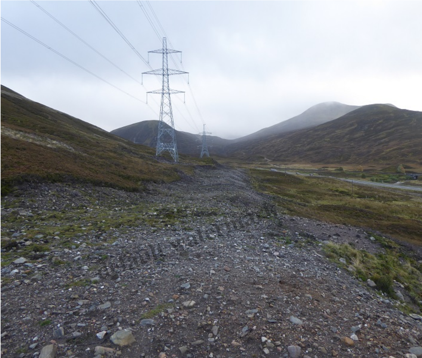
A section of “restored” track on the north Drumochter estate
