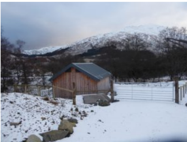
The much smaller Auchessan powerhouse
