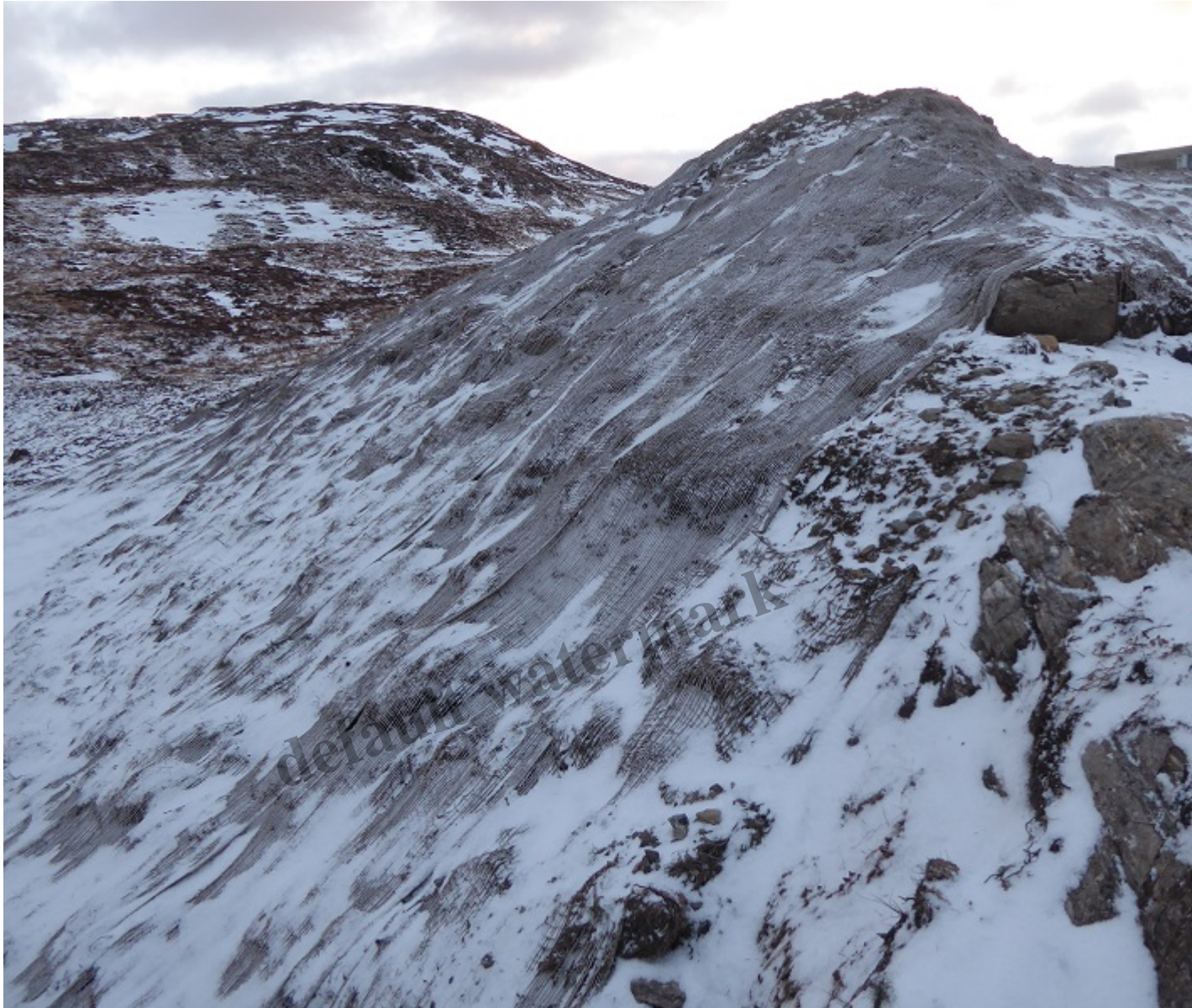
Mound of earth used to conceal intake from below
