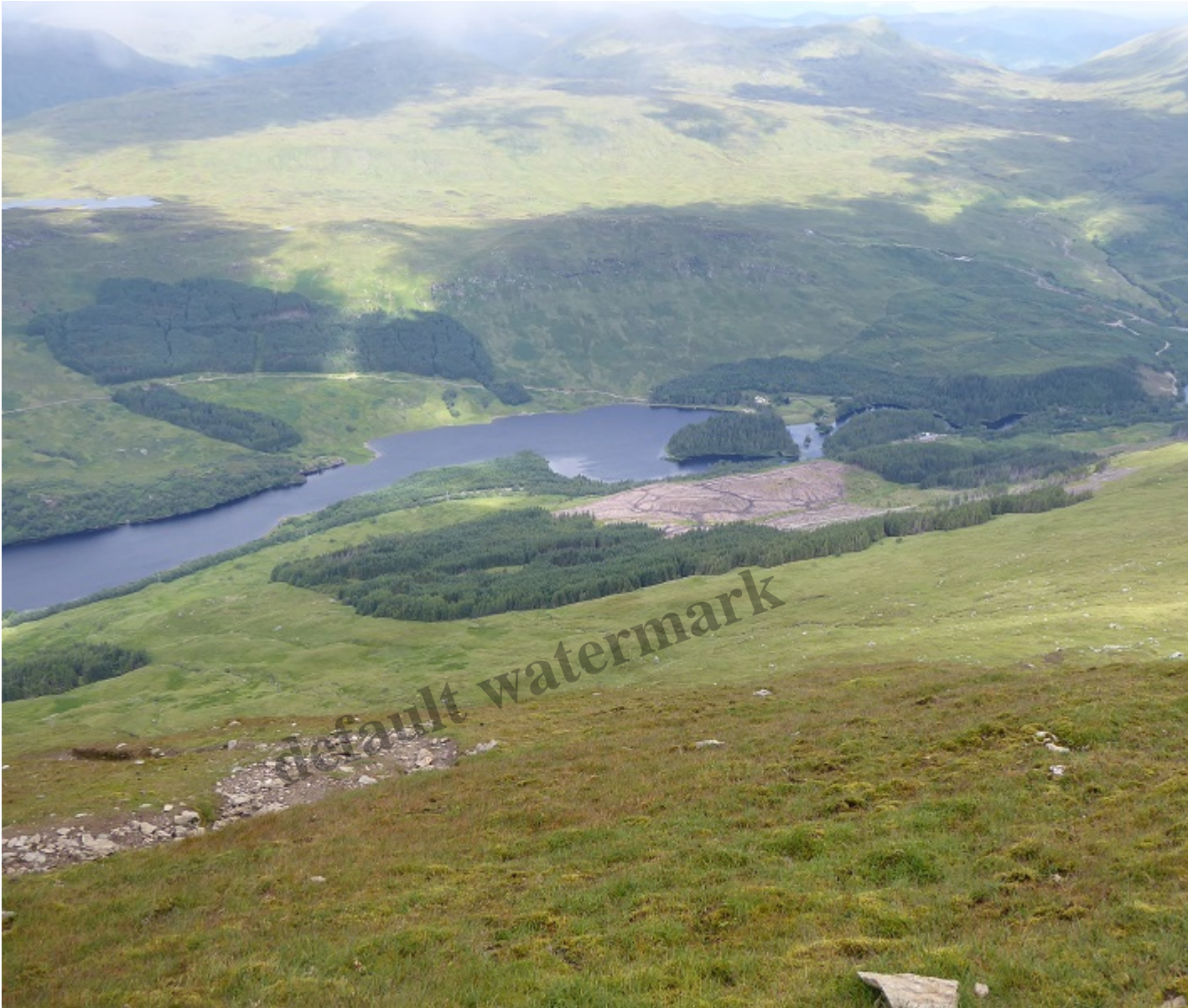
View of Allt Essan and Auchessan hydro tracks (right) from upper slopes of Ben More – note how the track basically follows the ridge and is therefore particularly prominent
