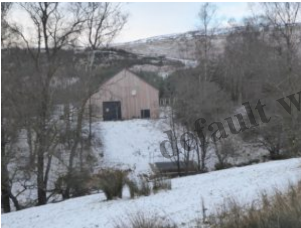
The Allt Essan powerhouse with the new intake track visible on hillside behind
