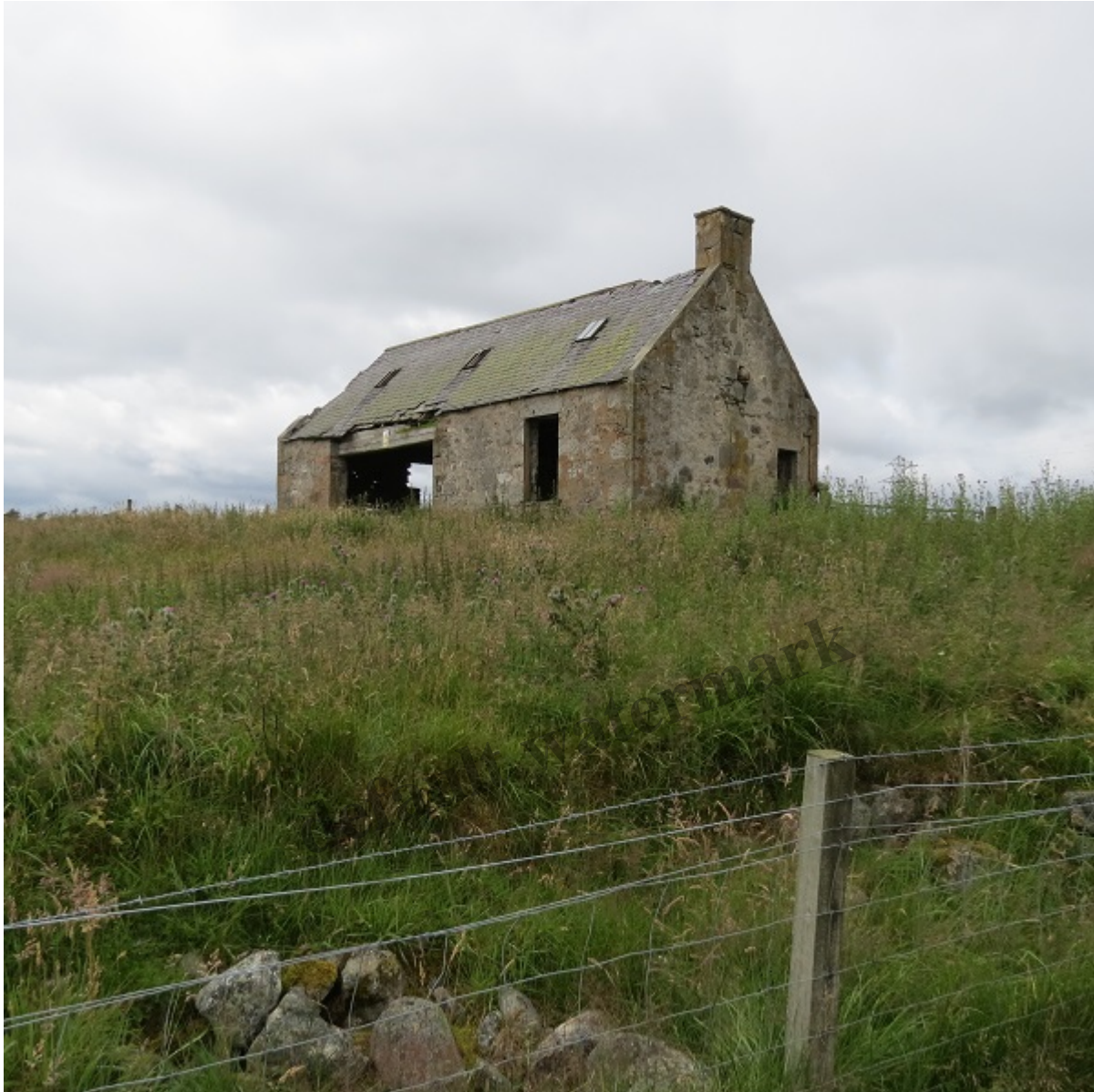
Derelict farm building, south of Kingussie and A9
