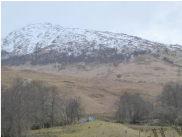
The Eas Eonan penstock below the A82, Ben Glas behind
