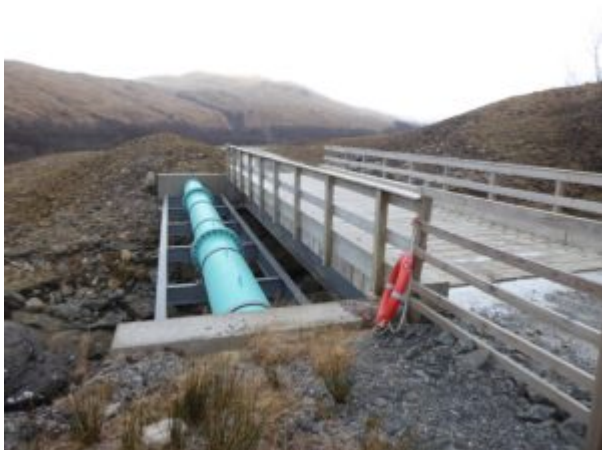
Allt Chuilinn penstock – according to Park guidance this should have been hidden UNDER the bridge
