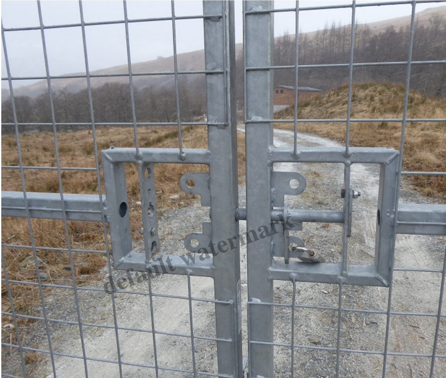
The padlocked gate
