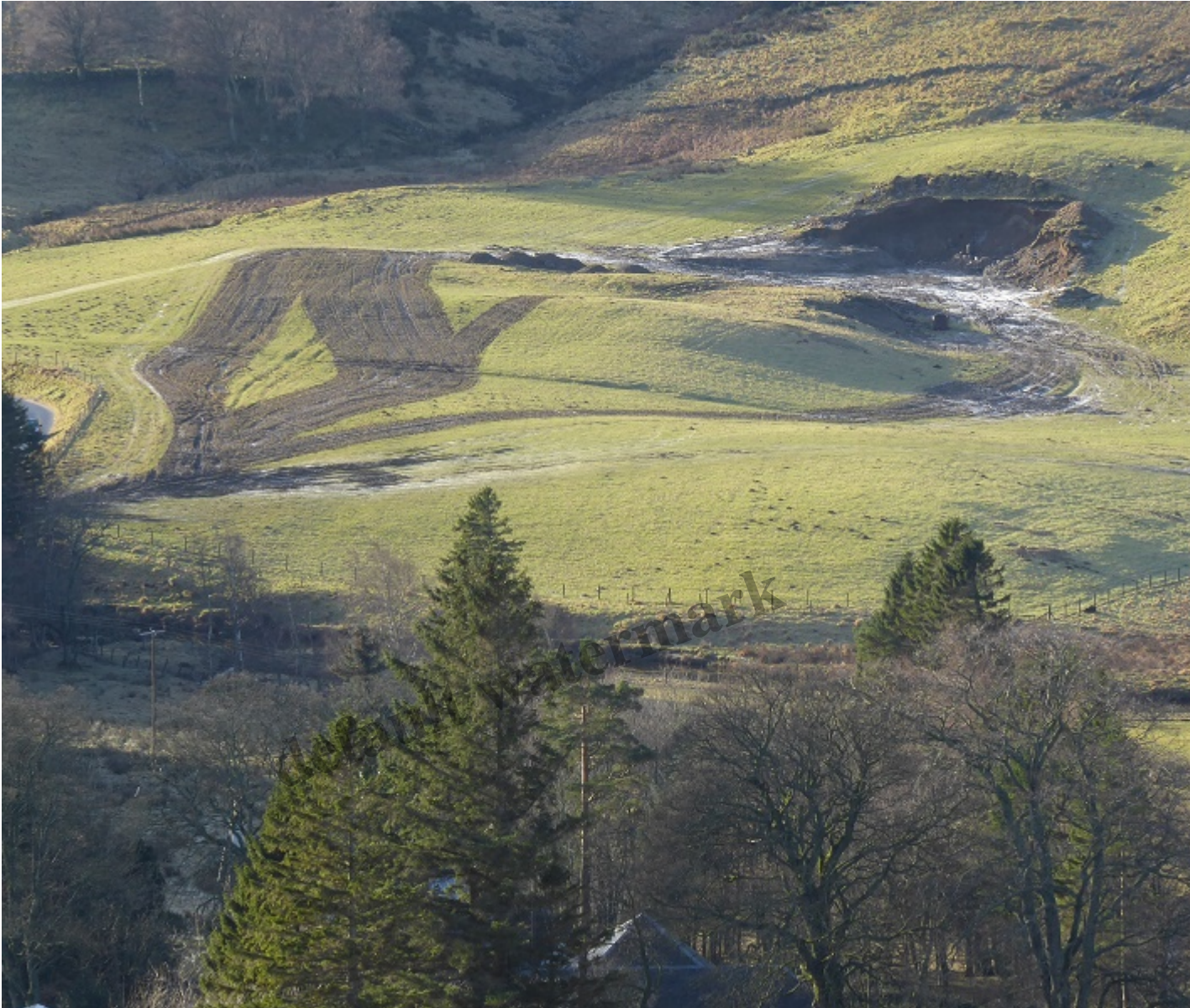
Earthworks opposite Glen Clova Hotel
