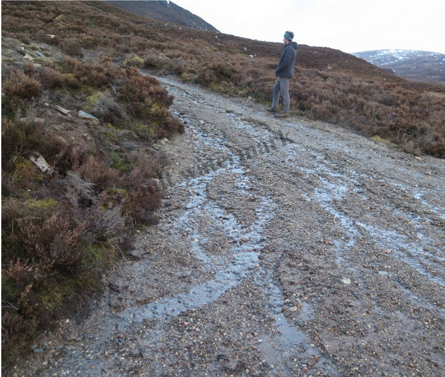
The new hill track at Glen Banchor above Newtonmore is already being seriously eroded. Photo Cre Morris
