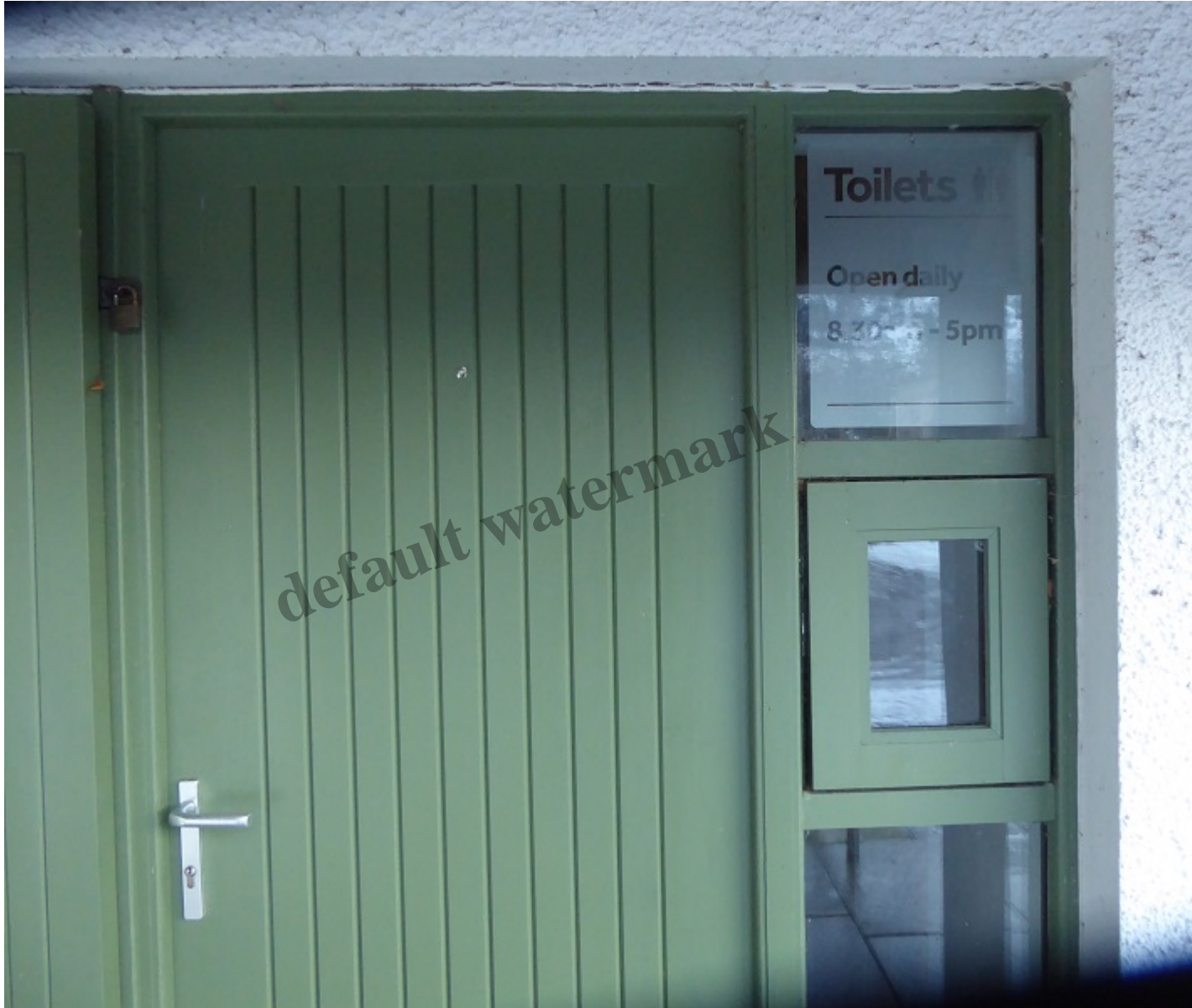
According to the notice the toilets should have been open 8.30-5pm
