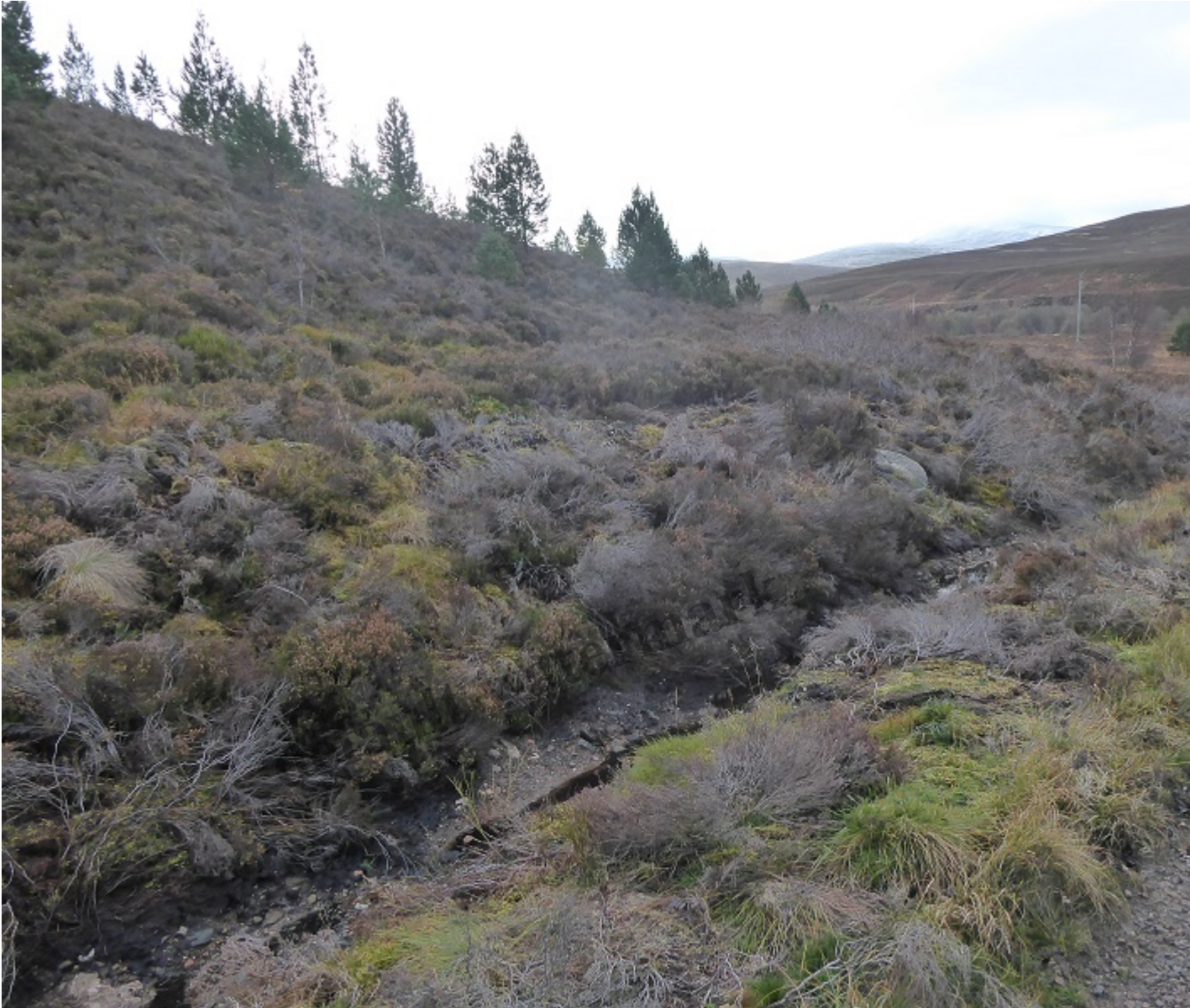
The buried cable is under the disturbed heather on the left side of the road
