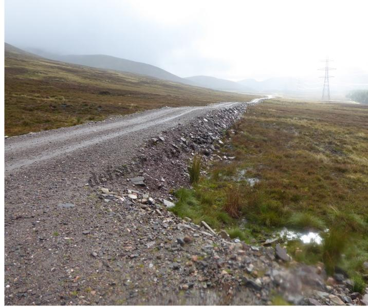
To construct this section of track Balfour Beatty as the main contractors allowed imported material to on the moor without any apparent attempt to save the vegetation beneath (there is no evidence of vebeing stored
