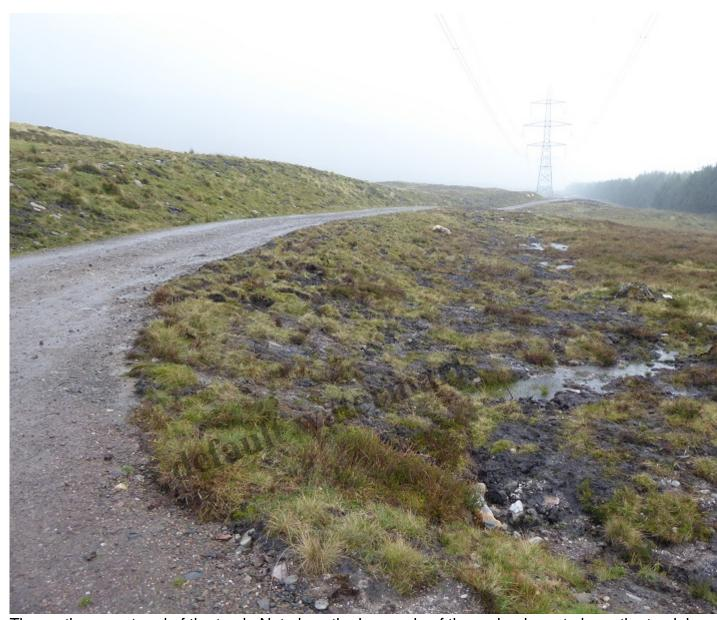
The northernmost end of the track. Note how the low angle of the embankment above the track has vegetation to recover quickly while stored turfs have been effectively used to restore the ground belotrack. October 2017.
