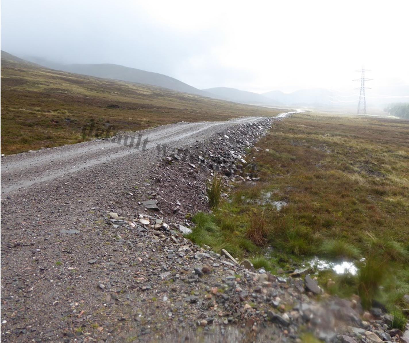
To construct this section of track Balfour Beatty as the main contractors allowed imported material to be dumped on the moor without any apparent attempt to save the vegetation beneath (there is no evidence of vegetation being stored
