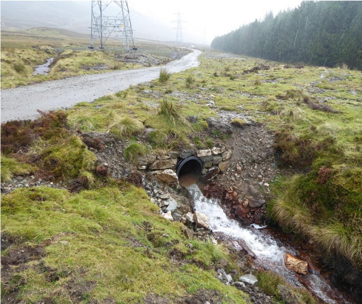
Before restoration, the track extended almost to the edge of the culvert. The bare banks on either side of the culvert appear the consequence of insufficient turf being stored for restoration purposes and are at high risk of erosion. October 2017.
