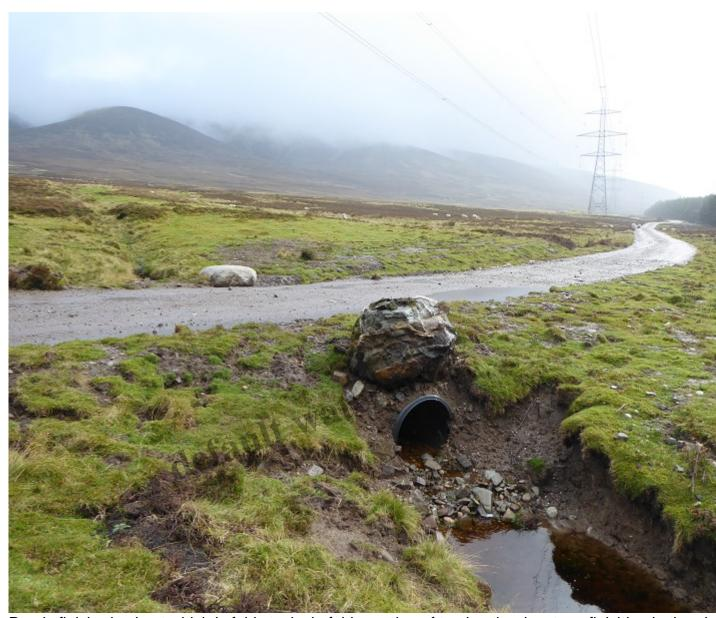
Poorly finished culvert which is fairly typical of this section of track – the dry stone finishing in the phowas the exception. Note the grouse tick mops in the background.
