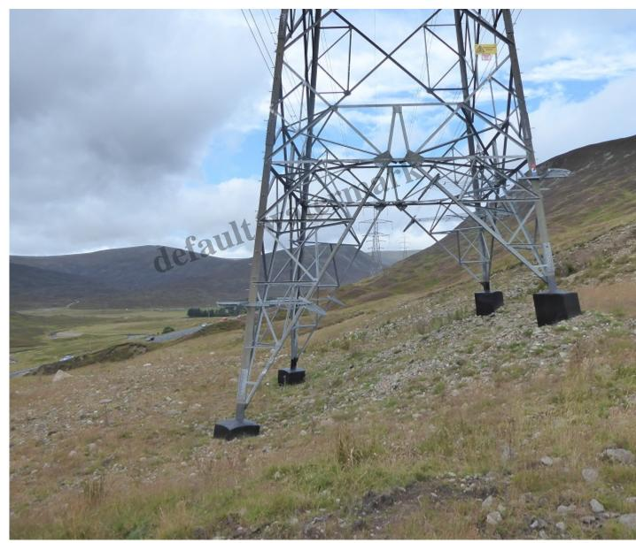
Tower south of Dalnaspidal. Some revegetation has taken place but because soils have been so dis not replaced properly grass and rush have replaced heather (as seen beyond the tower).
