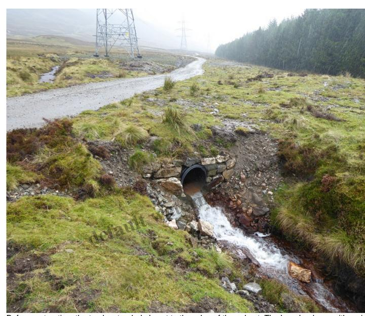
Before restoration, the track extended almost to the edge of the culvert. The bare banks on either side culvert appear the consequence of insufficient turf being stored for restoration purposes and are at he erosion. October 2017.
