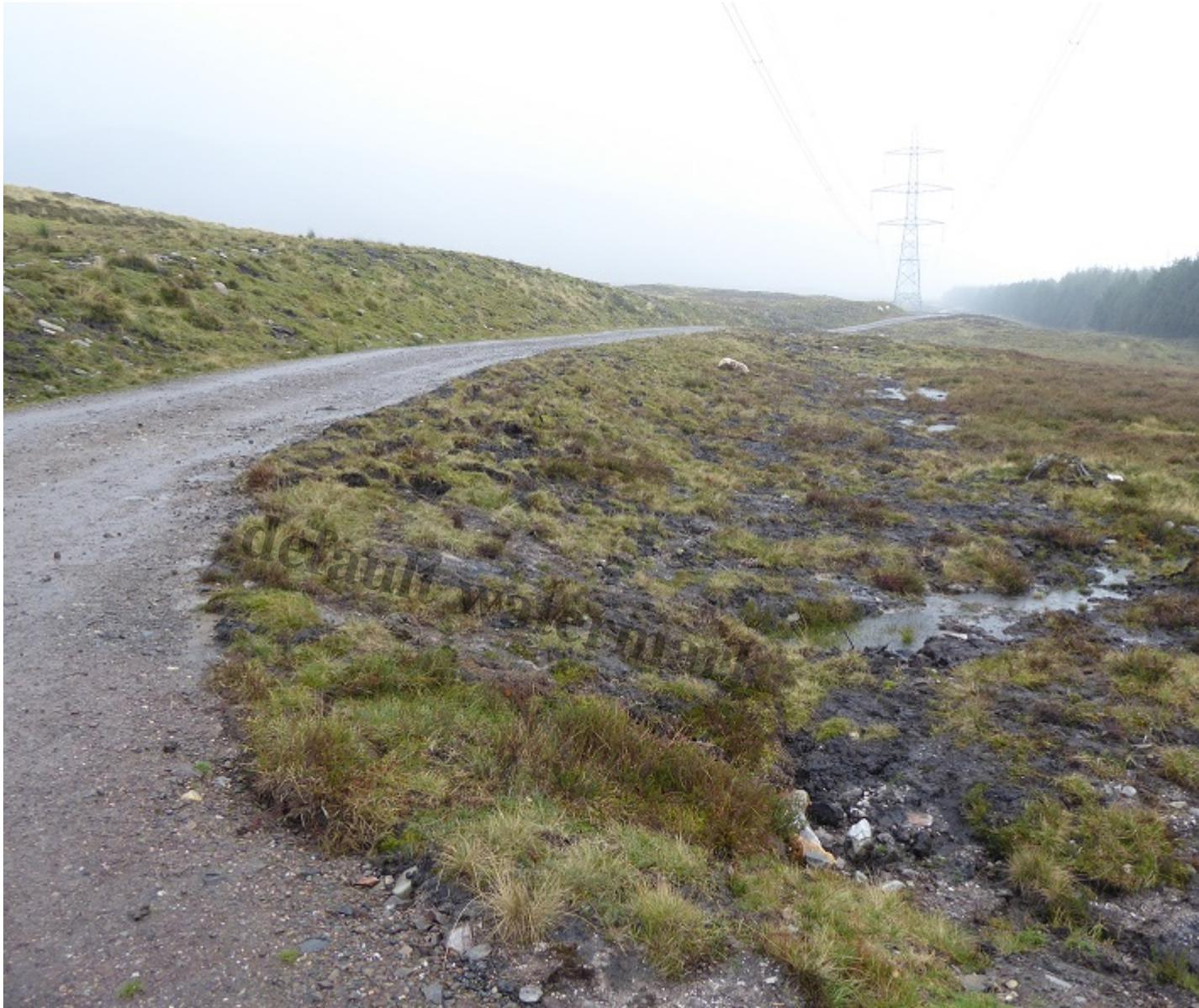
The northernmost end of the track. Note how the low angle of the embankment above the track has vegetation to recover quickly while stored turfs have been effectively used to restore the ground below. October 2017.
