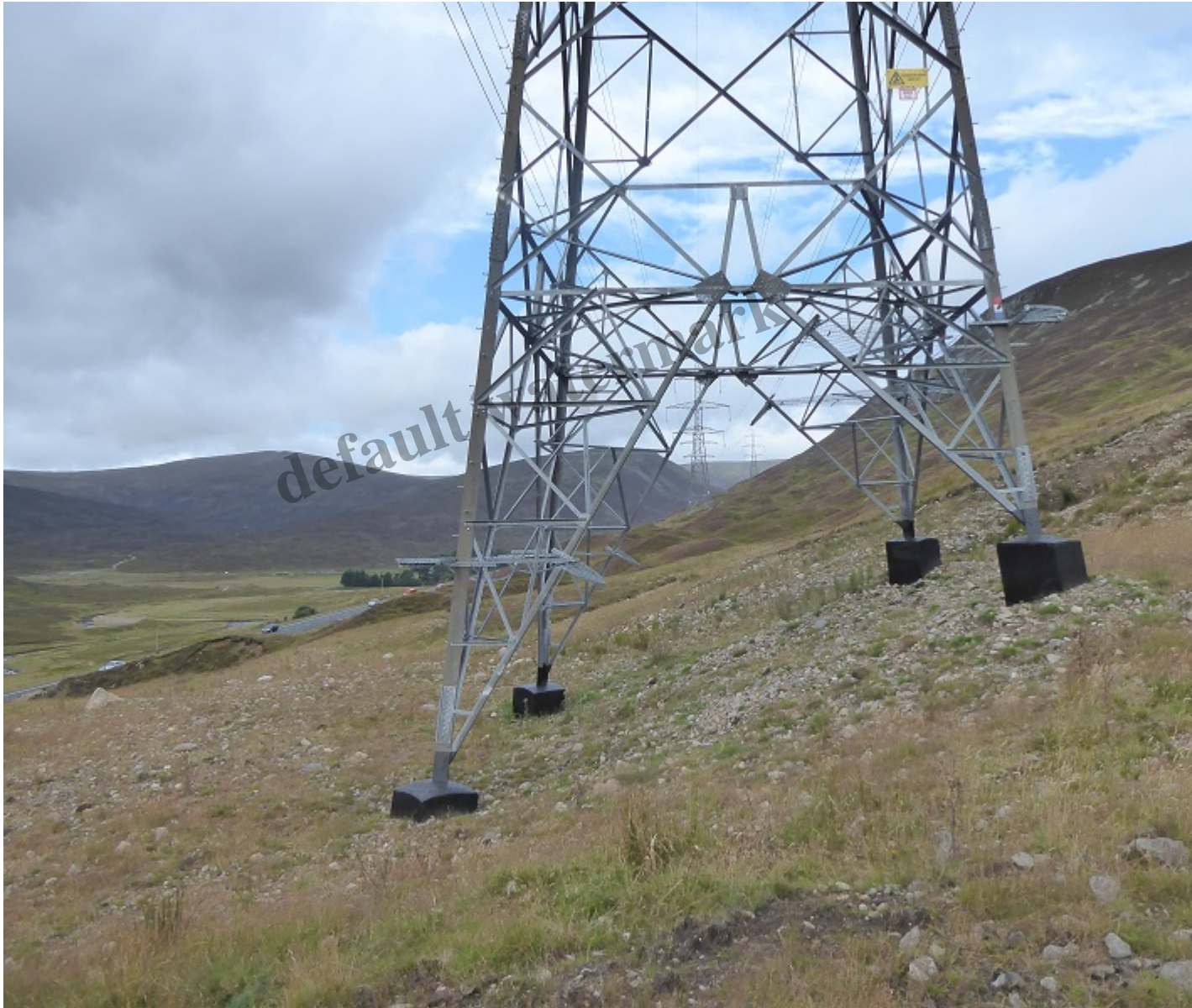
Tower south of Dalnaspidal. Some revegetation has taken place but because soils have been so disturbed not replaced properly grass and rush have replaced heather (as seen beyond the tower).
