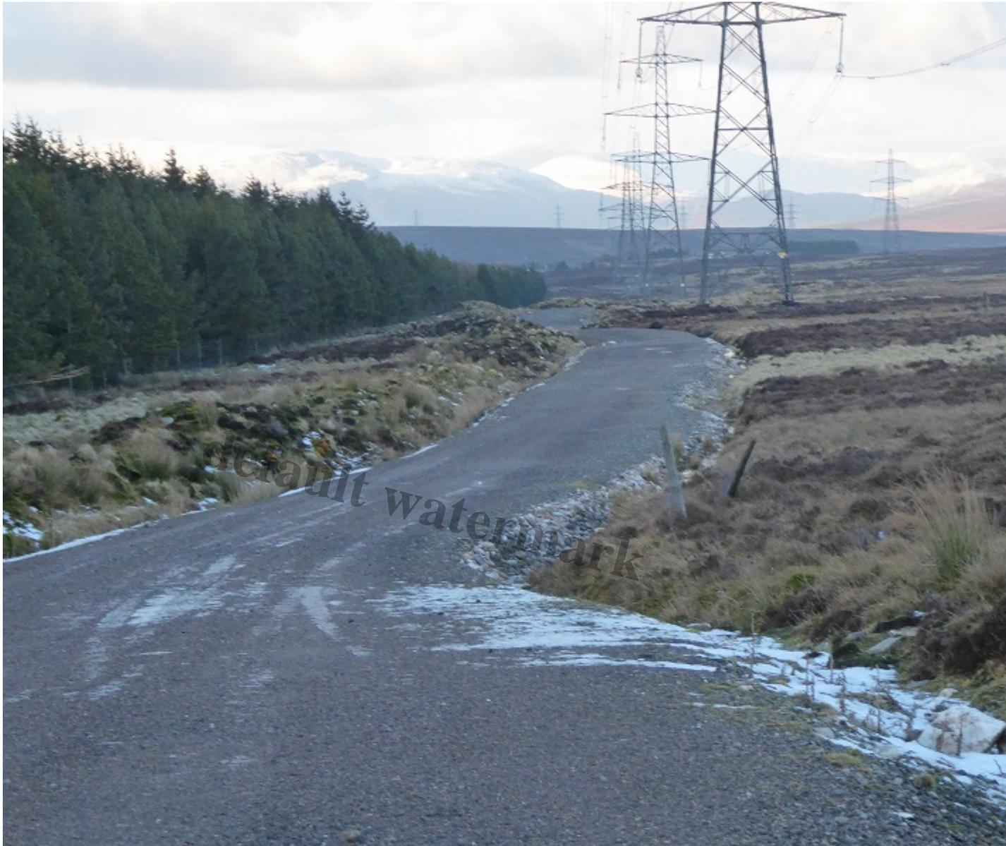
The start of the northern section of the Beauly Denny construction track (as indicated by arrow in map) as it appeared in February 2016. Note the ridge of vegetation covered spoil running along the left side of the track.
