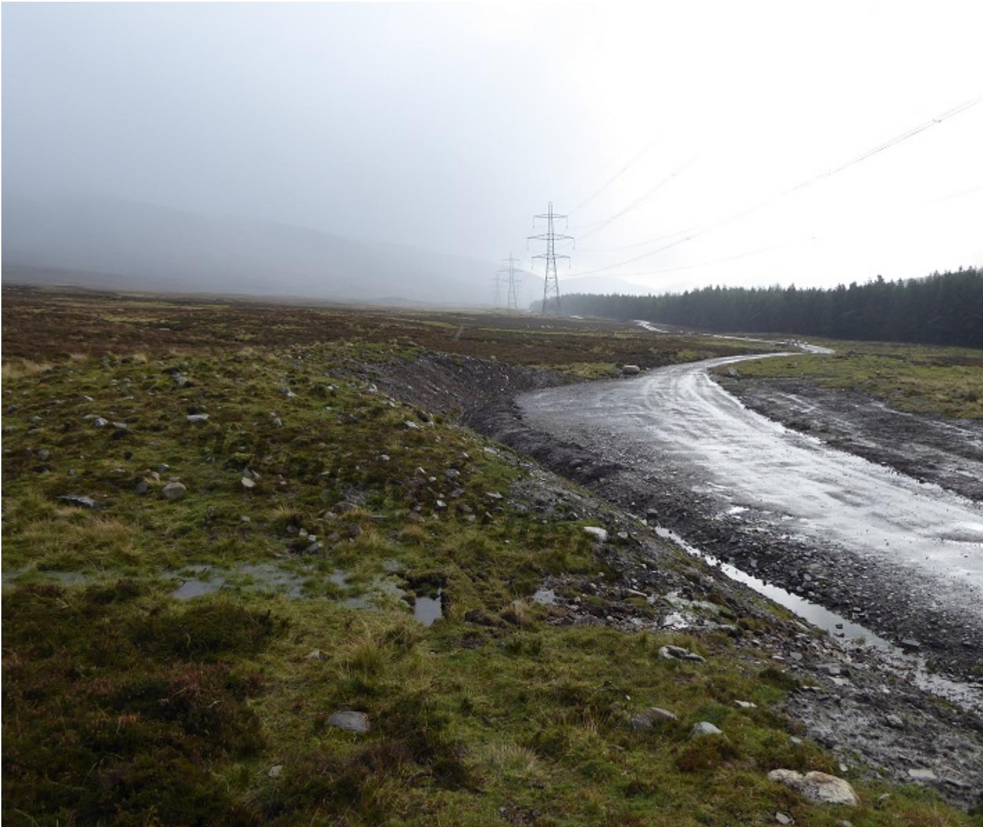
While generally the sides of the track have been well restored in places there appears to have been vegetation to do this: here there is an unvegetated section of ground to the right of the track while the unnecessarily large passing place appears to be another solution to this lack of material (which was responsibility).
