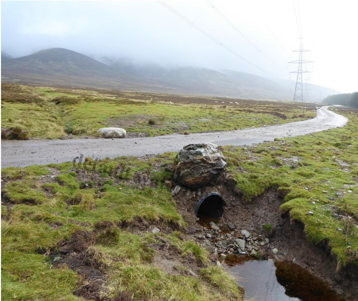
Poorly finished culvert which is fairly typical of this section of track â?? the dry stone finishing in the p was the exception. Note the grouse tick mops in the background.
