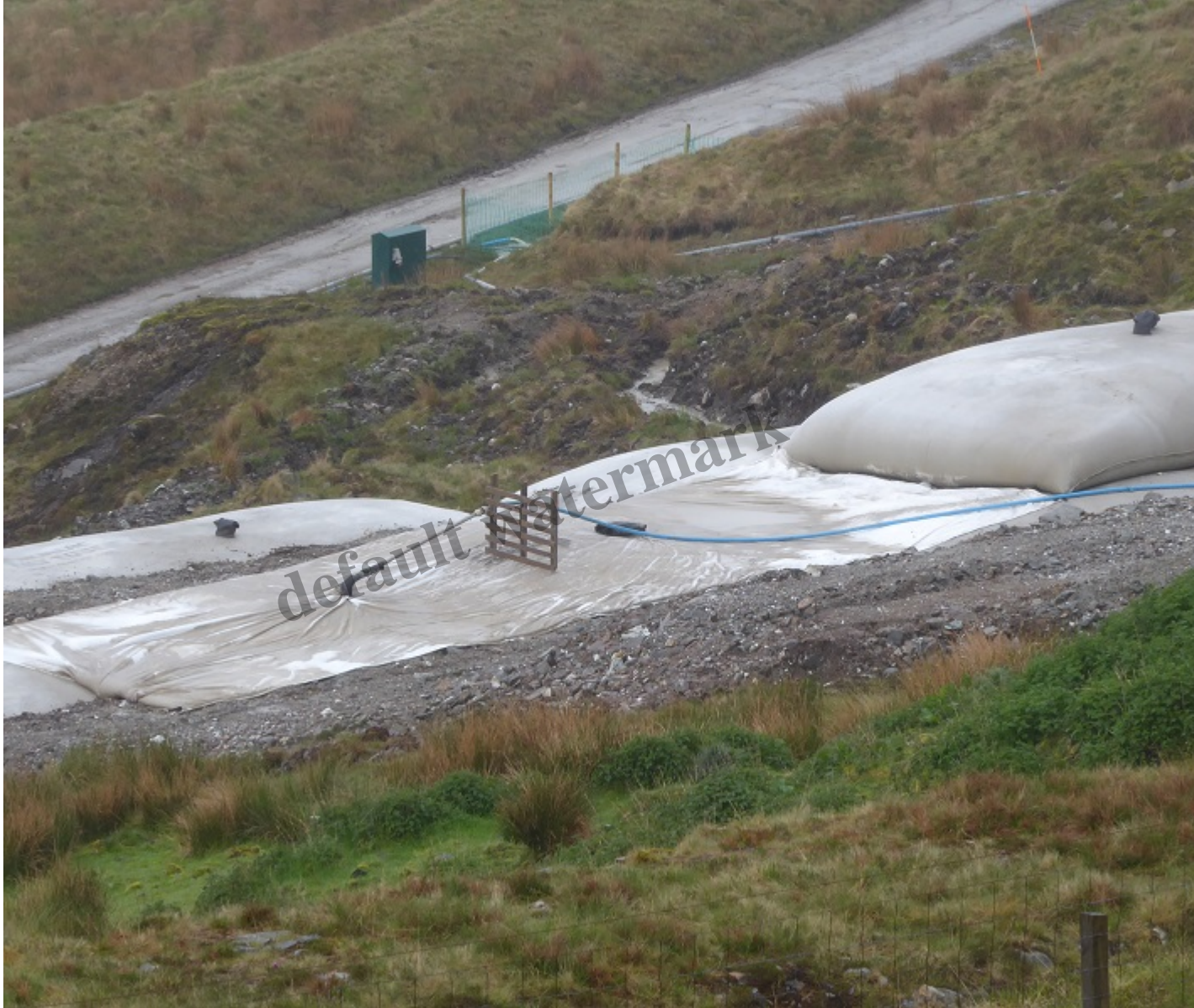
Filling of geotextile bags at Cononish – Photo Credit Nick Kempe
