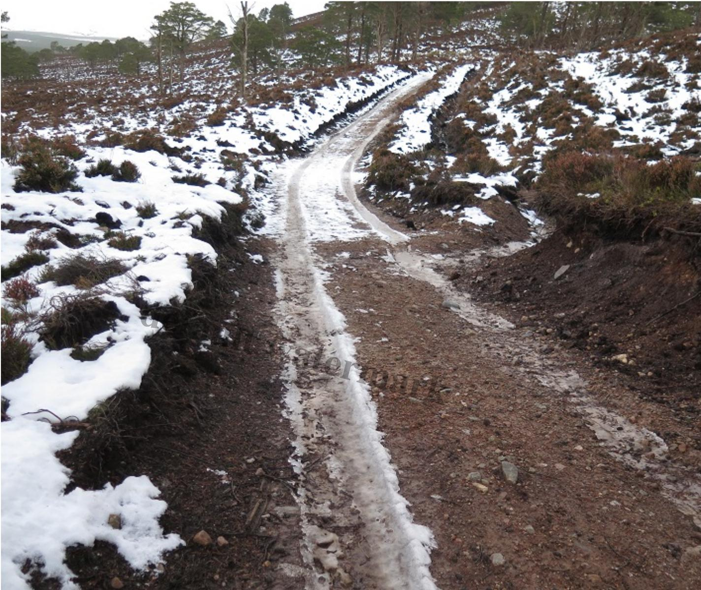
The track â?? a path formerly followed this line â?? appears to have been excavated with diggers and not finished, e.g the bank on the right and the drainage ditch beyond, is poor. Photo credit Dave Morris.
