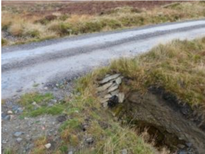
Finished culvert with turf placed above stone
