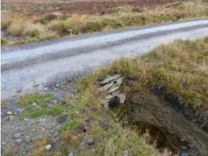
Finished culvert with turf placed above stone
