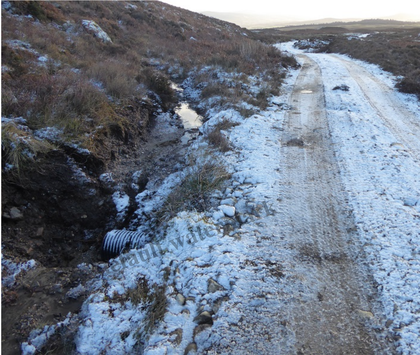
Unfinished culvert and new drainage ditch
