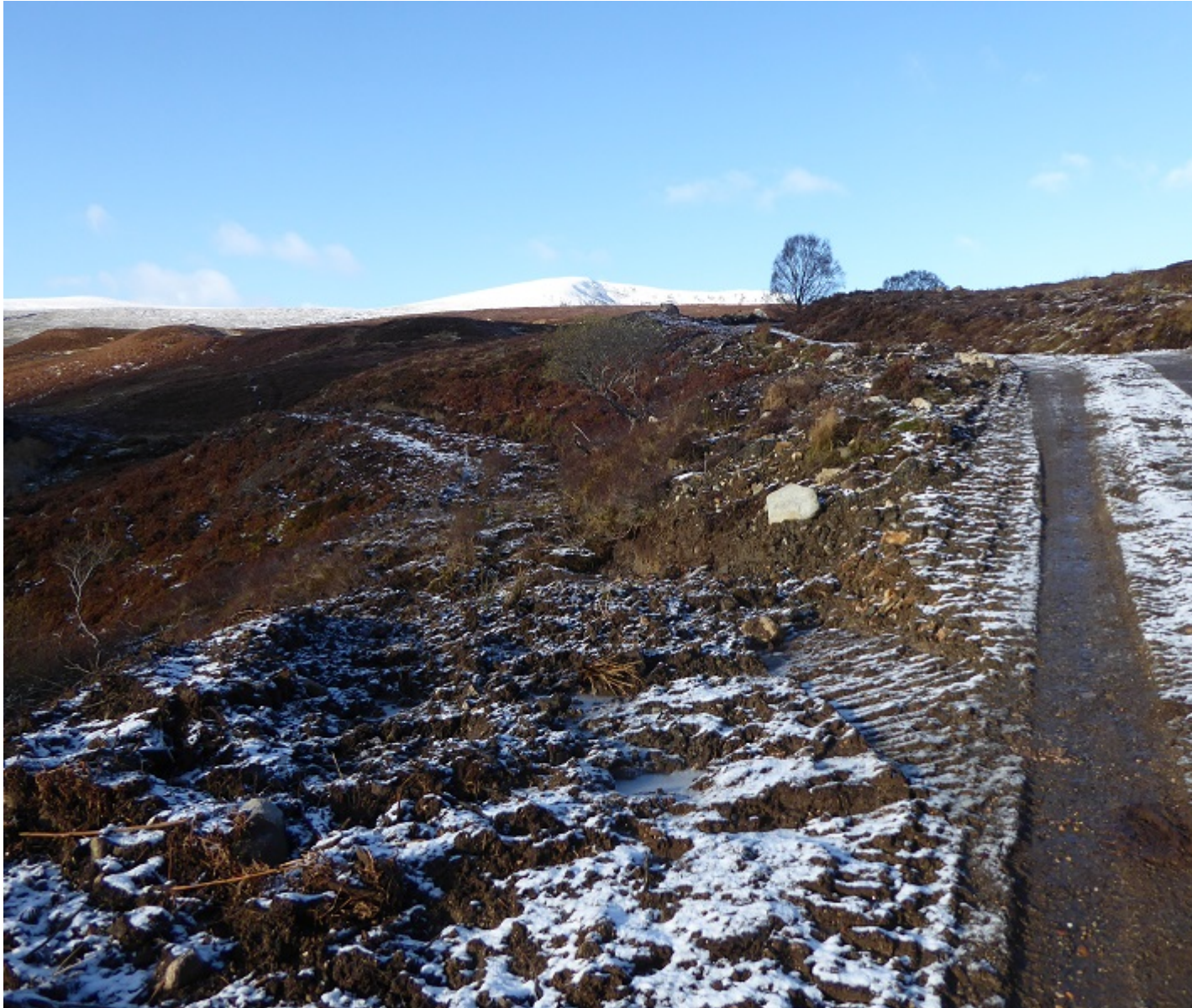
The edge of the existing track appears to have been excavated to facilitate ATV access to land on the other side of the road, creating a new track
