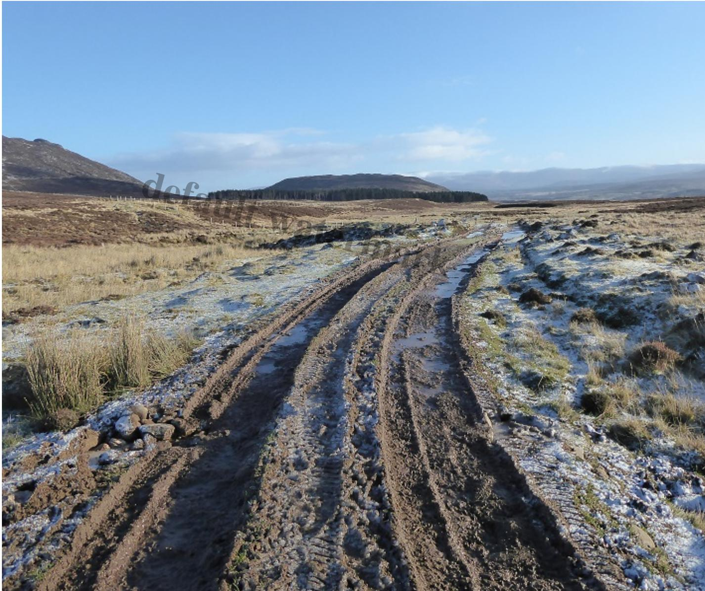
Looking back along the Allt na Beinne track to the central Cairngorms. The movement of heavy vehicles on the track in wet conditions has caused significant damage and helped destroy its quality as a recreational area.
