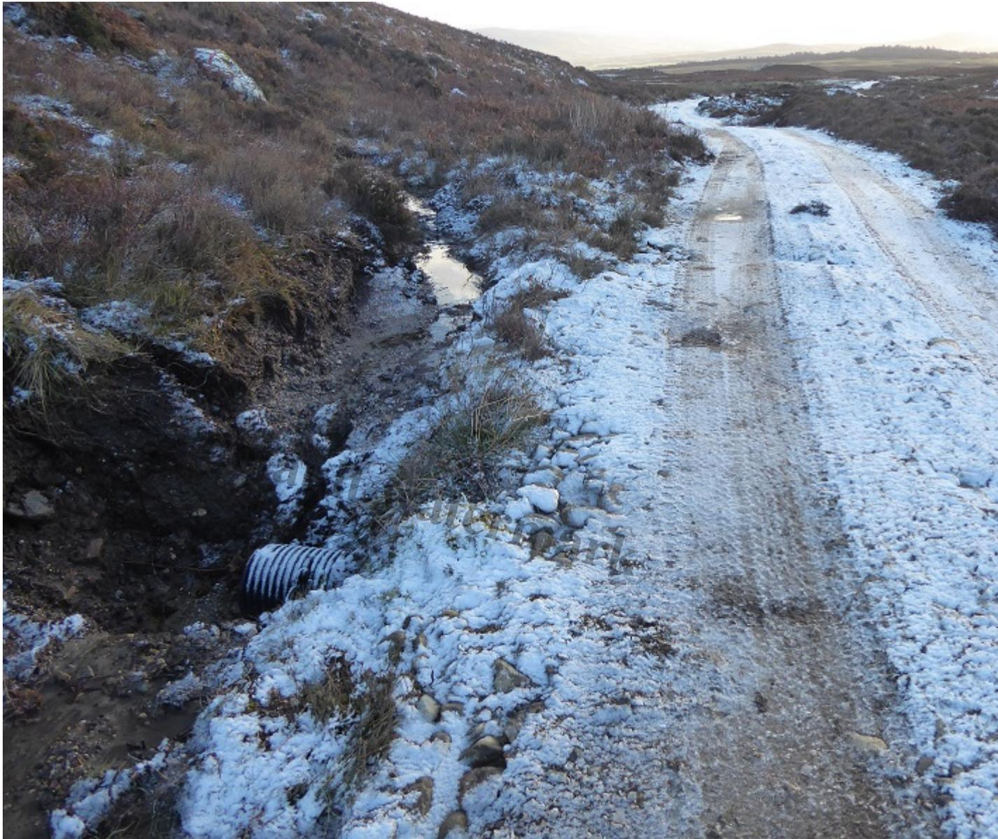
Unfinished culvert and new drainage ditch
