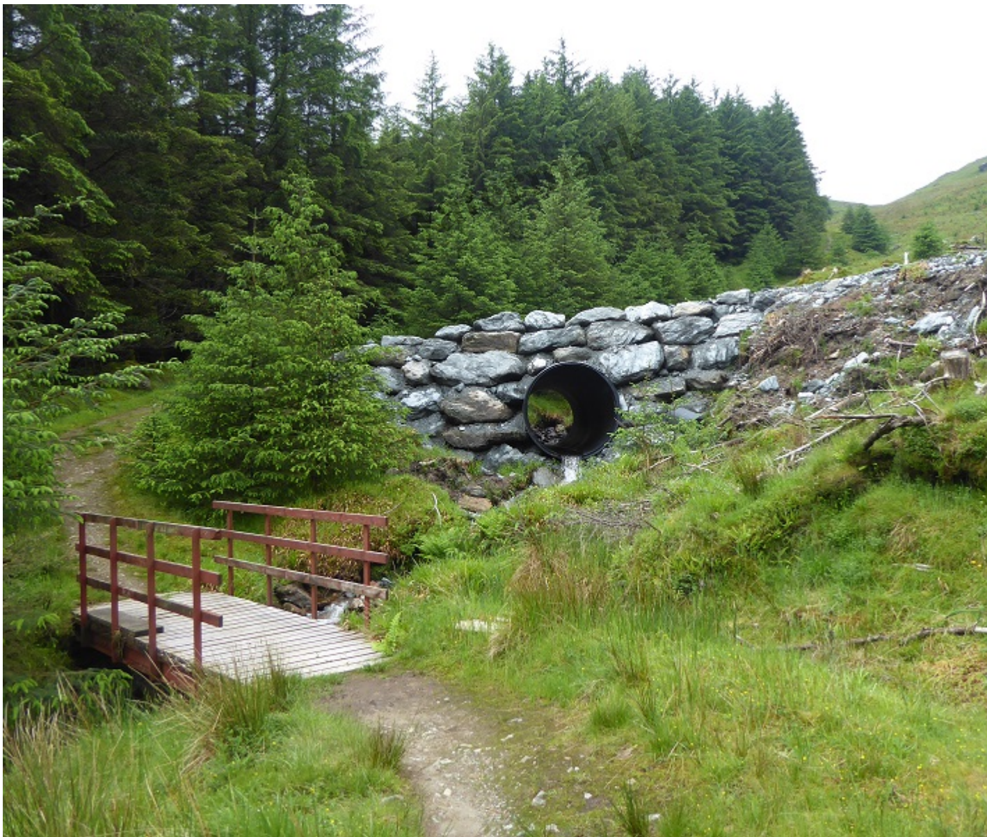
View of track extension from below
