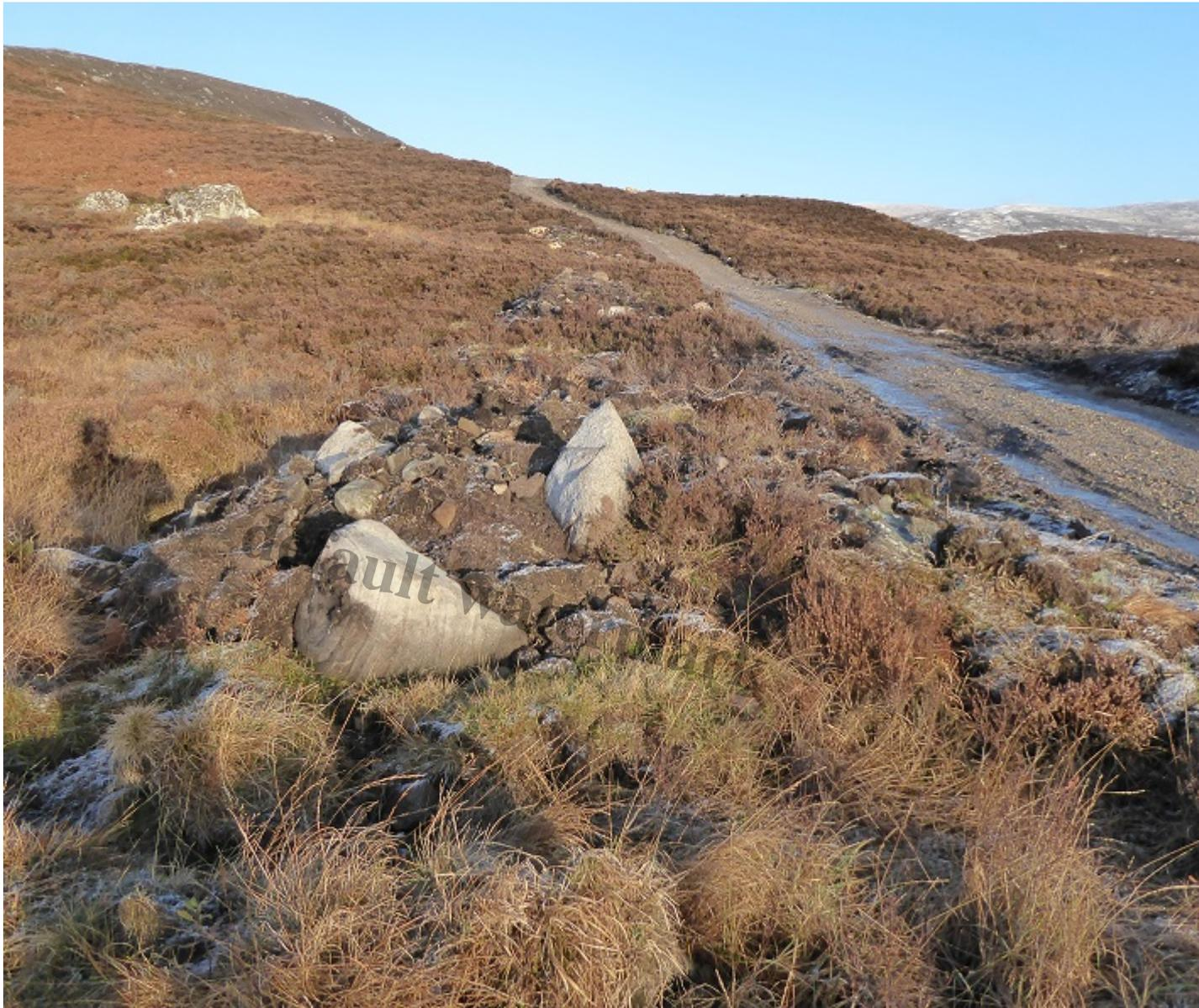
There is evidence all along the former landrover track that major upgrading works have taken place. Large lumps of turf in the foreground which could have been replaced down the centre of the track reduce erosion and the landscape impact.
