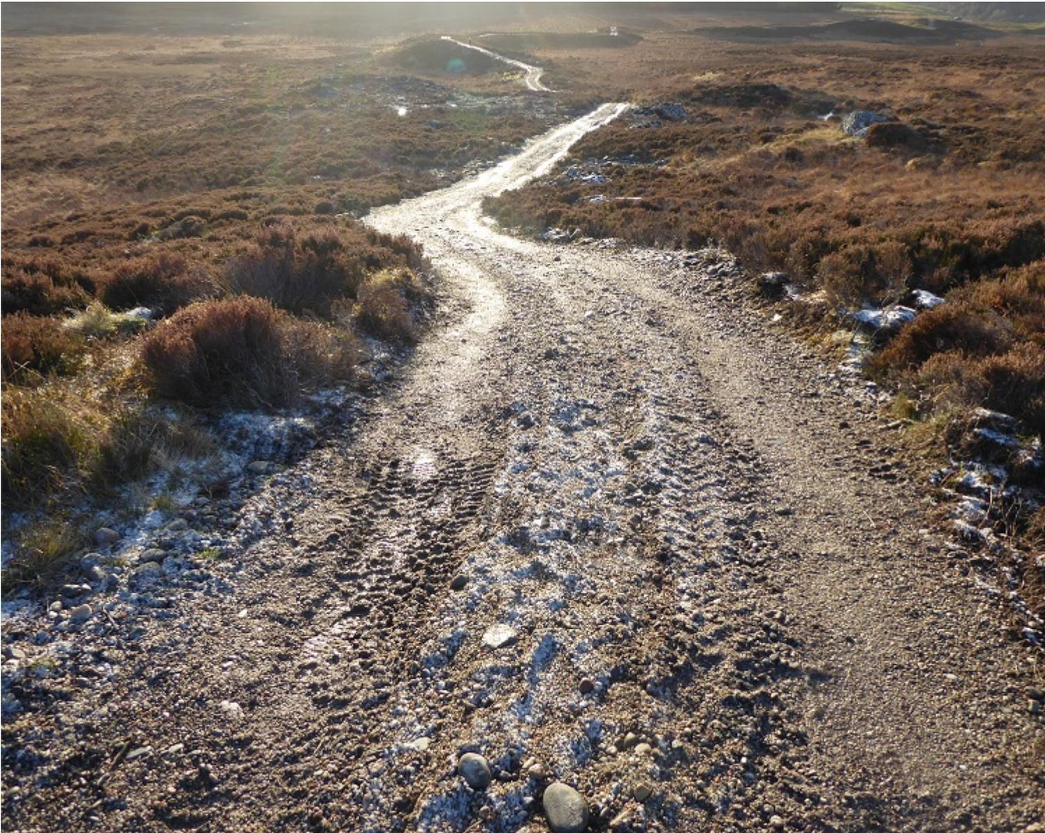
The upper section of the track is too steep and already eroding away, not helped by the lack of vegetation down the middle and an absence of drainage bars which means water runs straight down the line of the track.
