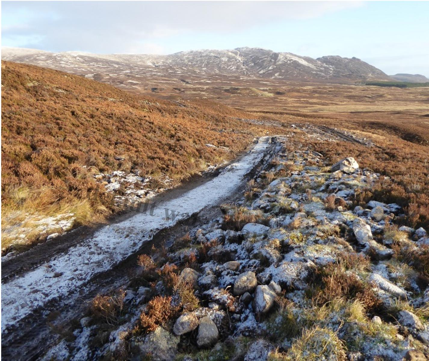
The new track contours round and down the hillside from just below the sheep holding area. You can see the excavated boulders and vegetation dumped on the right of the track.
