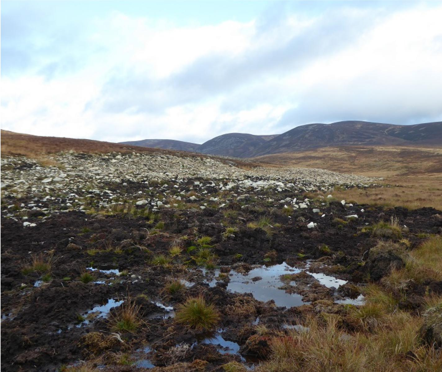
The start of the section of unrestored pipeline marked by the boulder field. Note the large peat turves far right which appear to date from original excavation and have never been used for restoration purposes.
