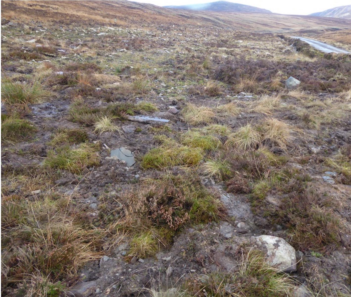
Restored boulder band scar showing how “robbed” turves and soil have been used.
