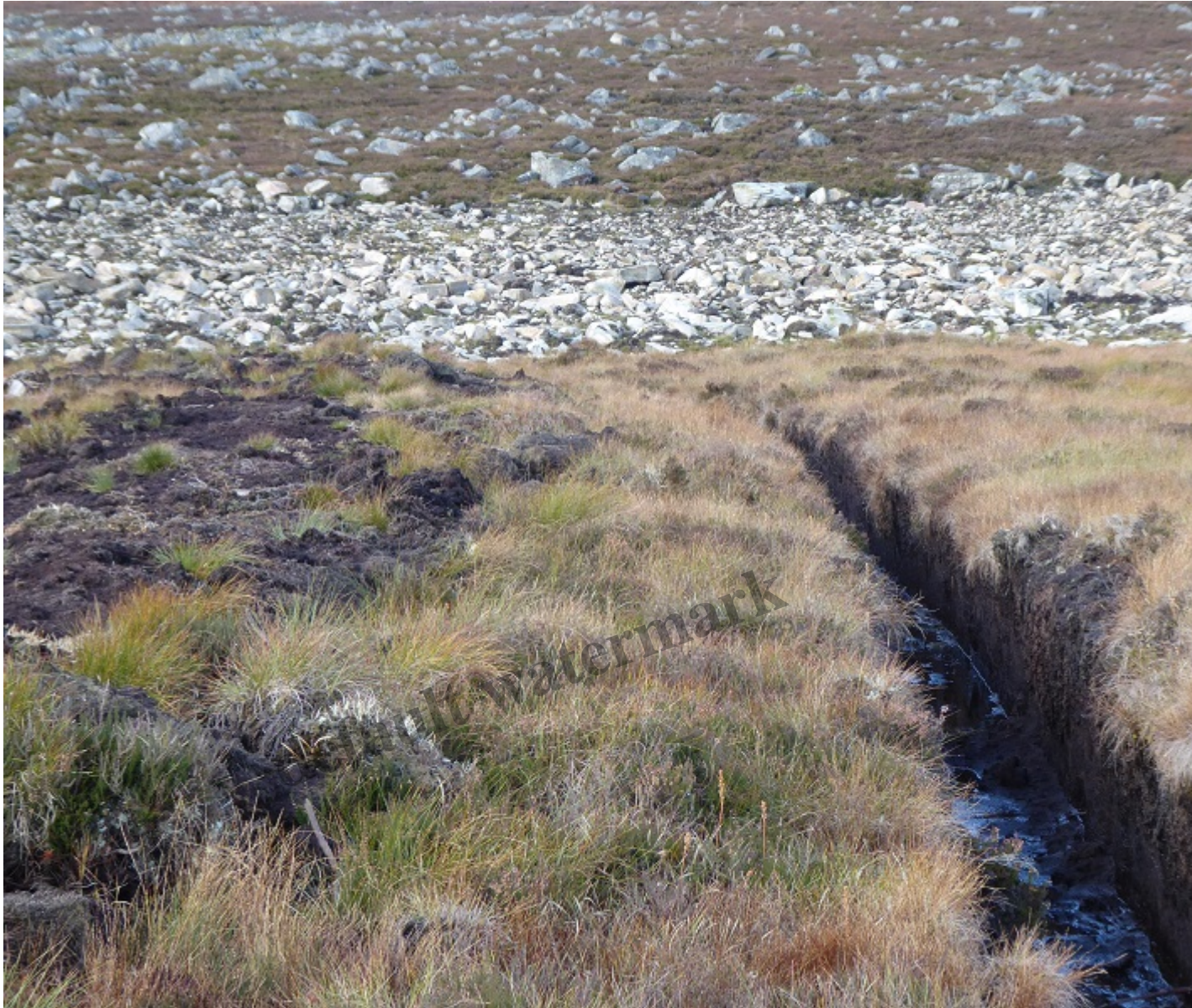
New drainage ditch showing depth of peat. The excavated material has been dumped on left.
