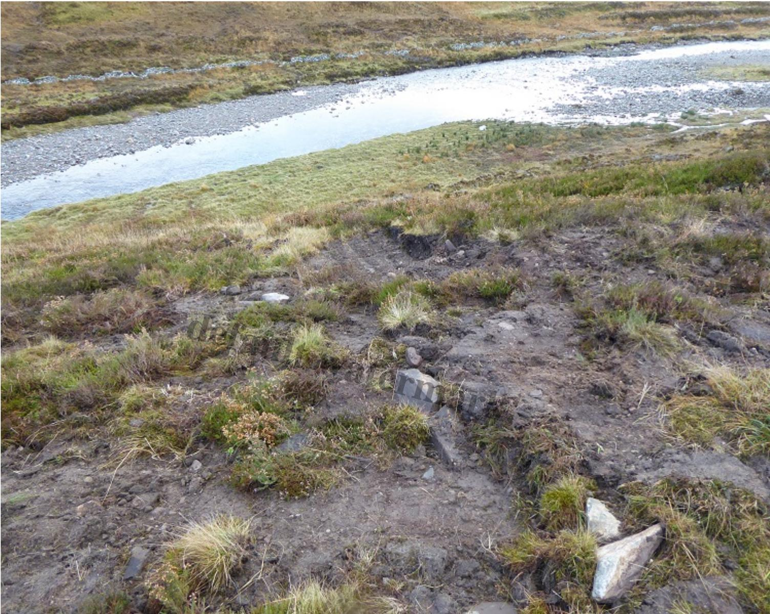
Photo showing how turves and other vegetation has been “robbed” from below the track to cover up the scar above. Note the digger scoop mark centre. [/caption]
