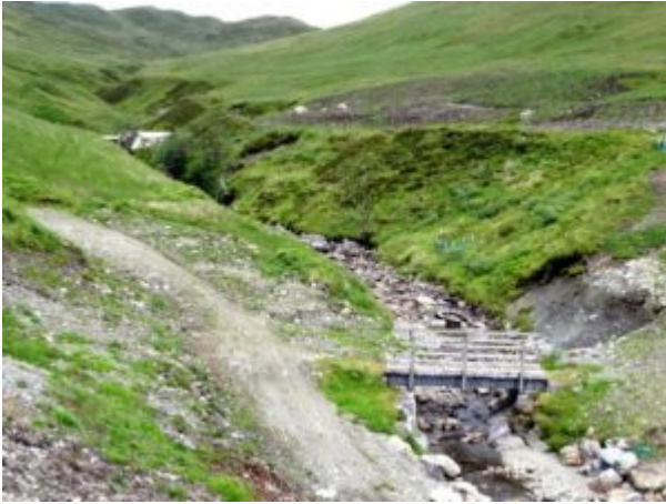
The main intake is well hidden
