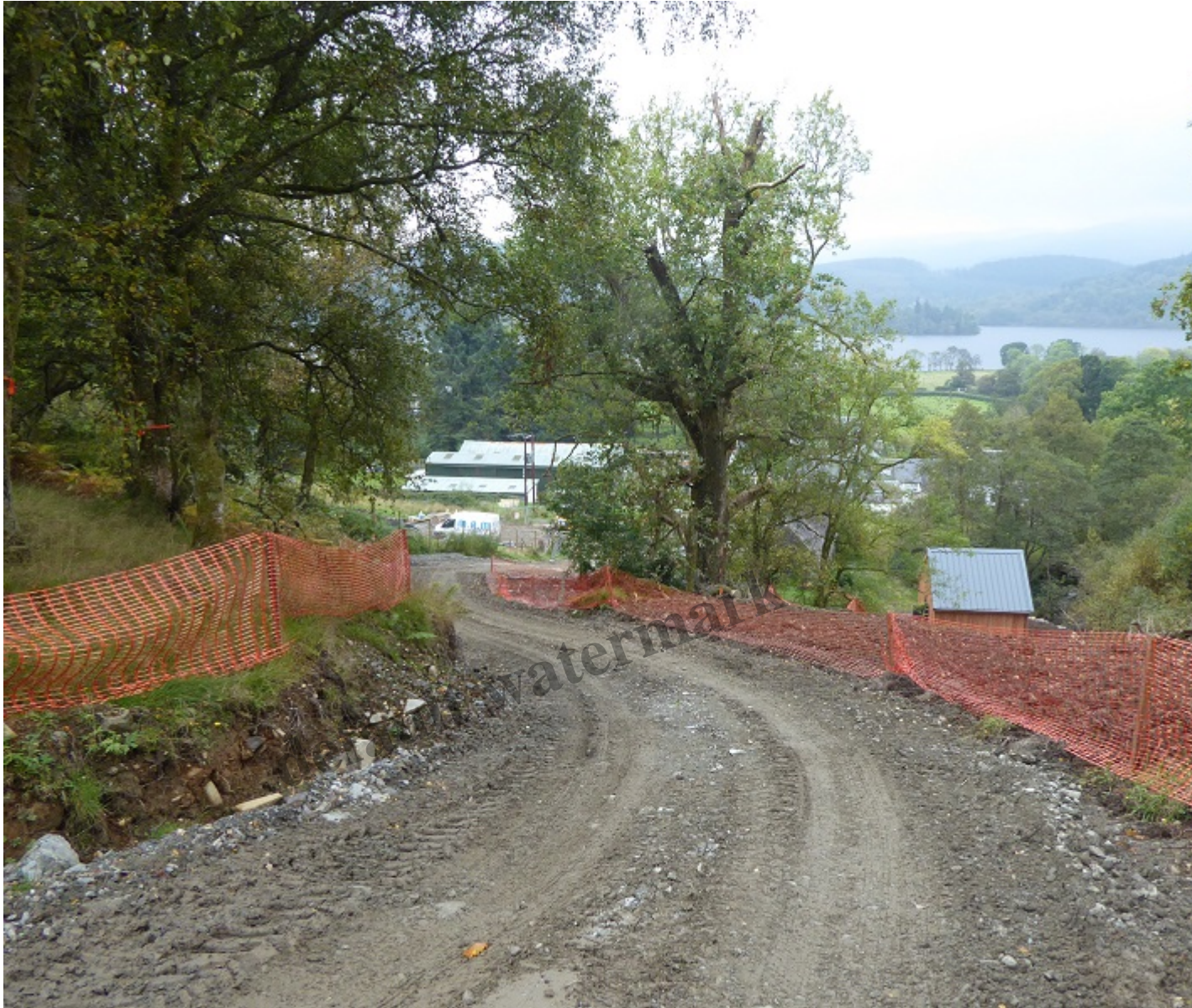
Powerhouse is wooden building right of centre
