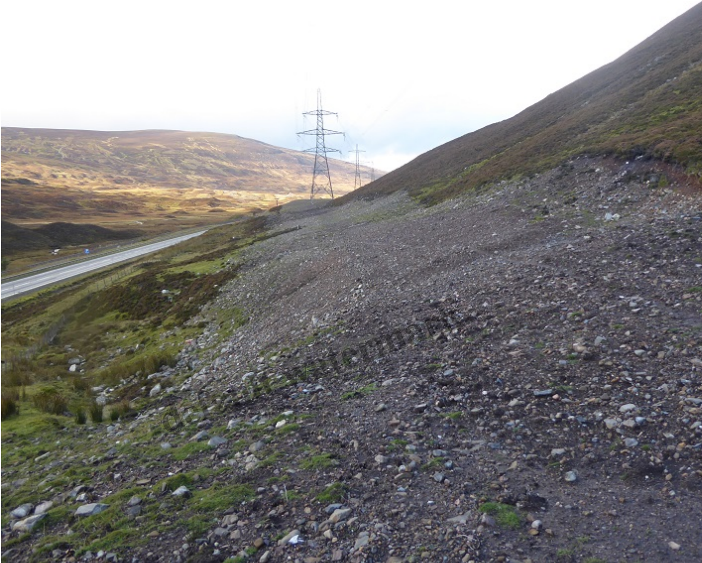
Section south of previous photo looking north
