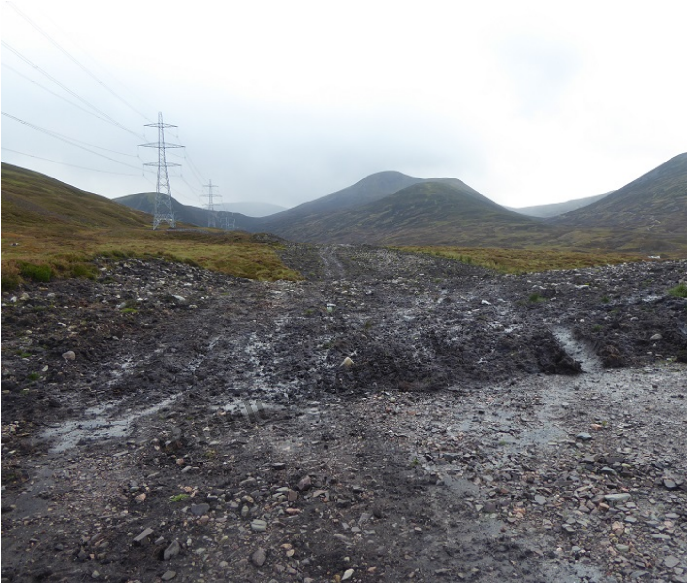
The boundary between the unrestored section of track just south of North Drumochter Lodge policy v and the restored section.
