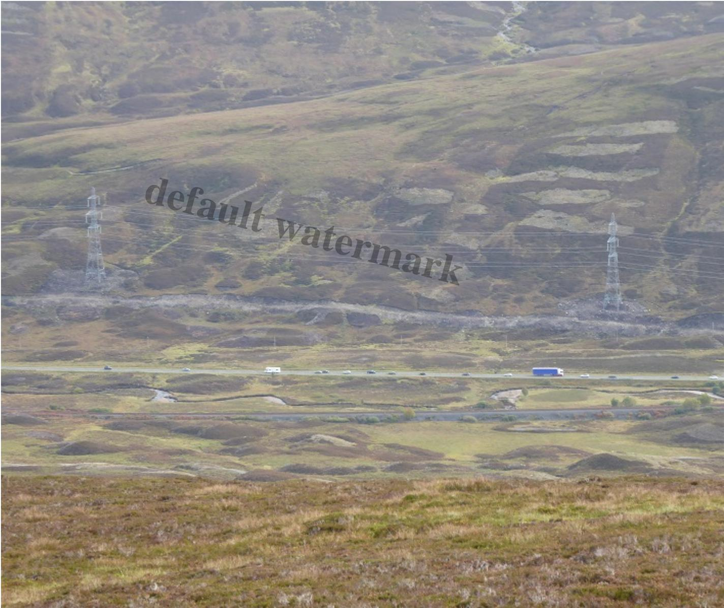
The “restored” construction track just south of Balsporran Cottage forms a gash across the hillsides. The track will remain highly visible even if the vegetation does recover because the “bench” which was cut across the hillside by cut and fill construction to provide a flat track has not been re-landscaped.
