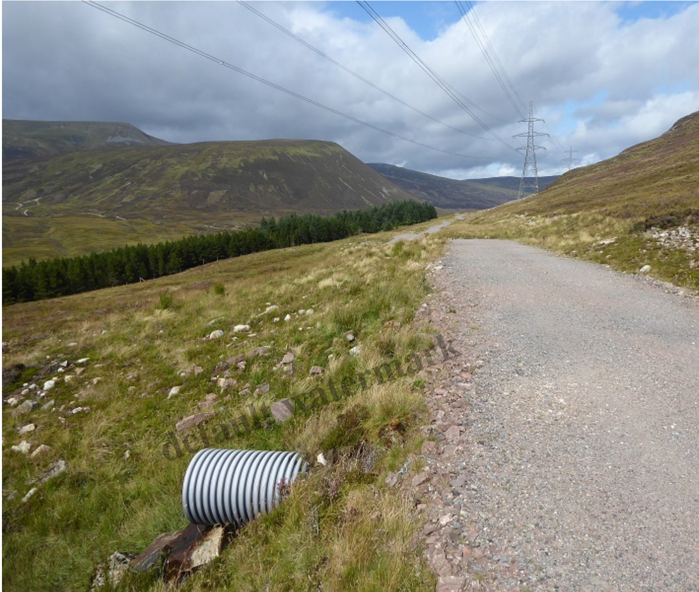
There are relatively few protruding culverts but more would appear if the track had been narrowed
