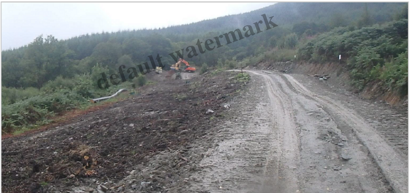
Photo 7: upper section of track at about 105mm elevation looking north west
