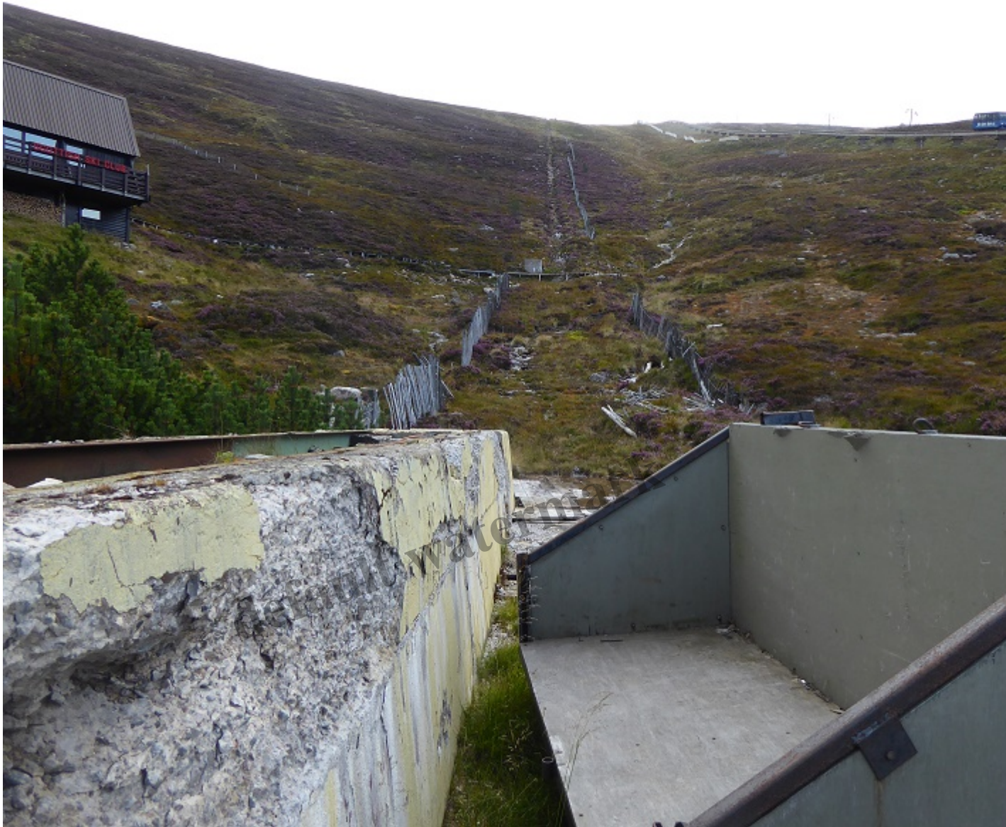
The former White Lady t-bar base and associated mess as it appeared in August 2017 can clearly be seen from the funicular (top right).
