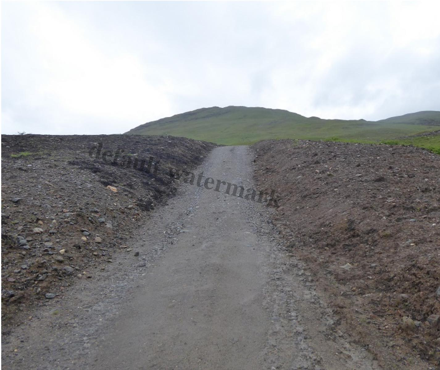
Bare ground all along the track results from the failure of the LLTNPA to enforce the planning conditions that require the turf be retained and stored properly.
