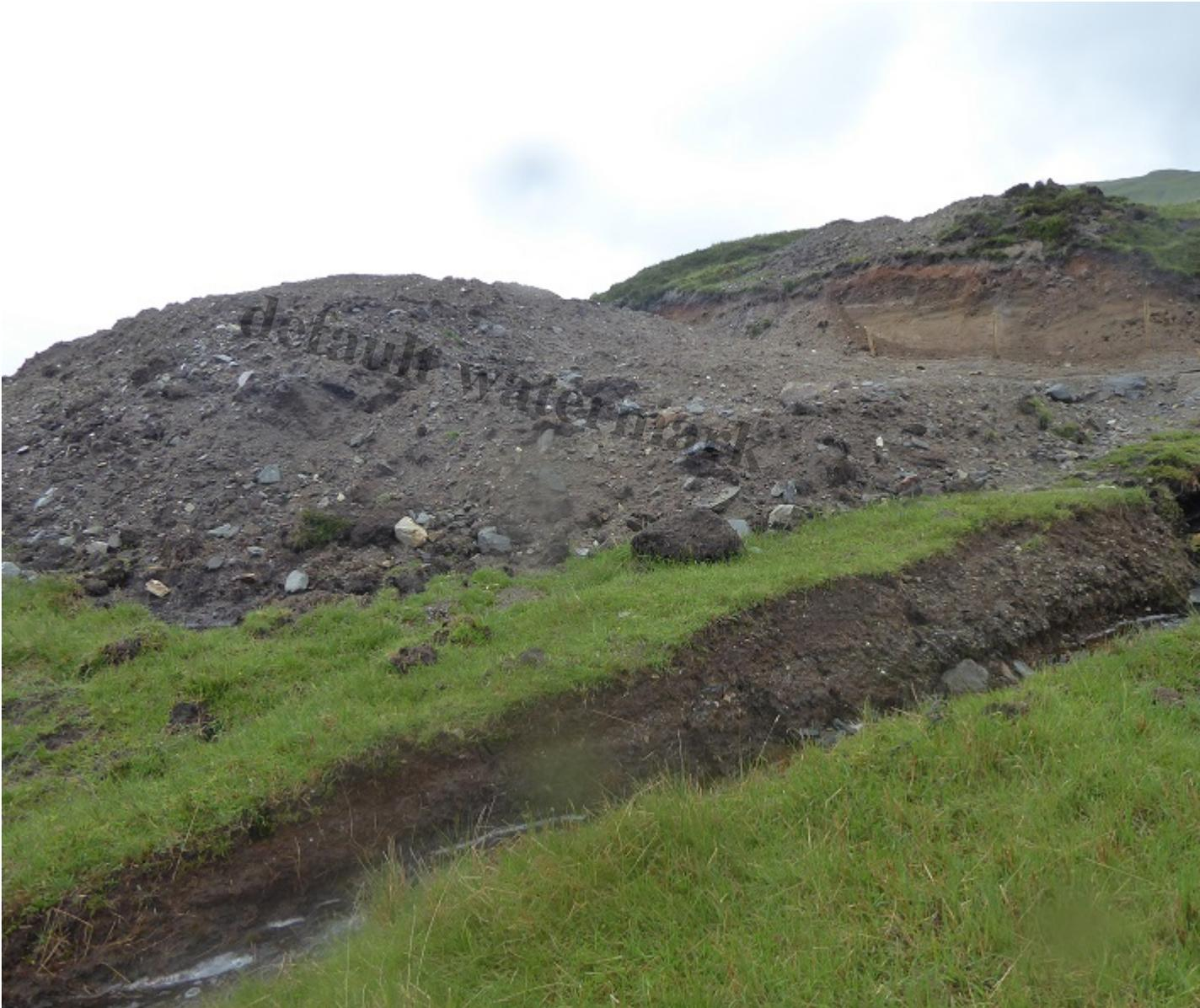
A example of the destruction created by the Ledcharrie track. The slope above the track is too steep so spoil has been dumped below it without any sign of re-landscaping. The contractor had removed all signs of the track from the site indicating the Developer, Glen Hydro Development Ltd, saw this as the "finished product".
