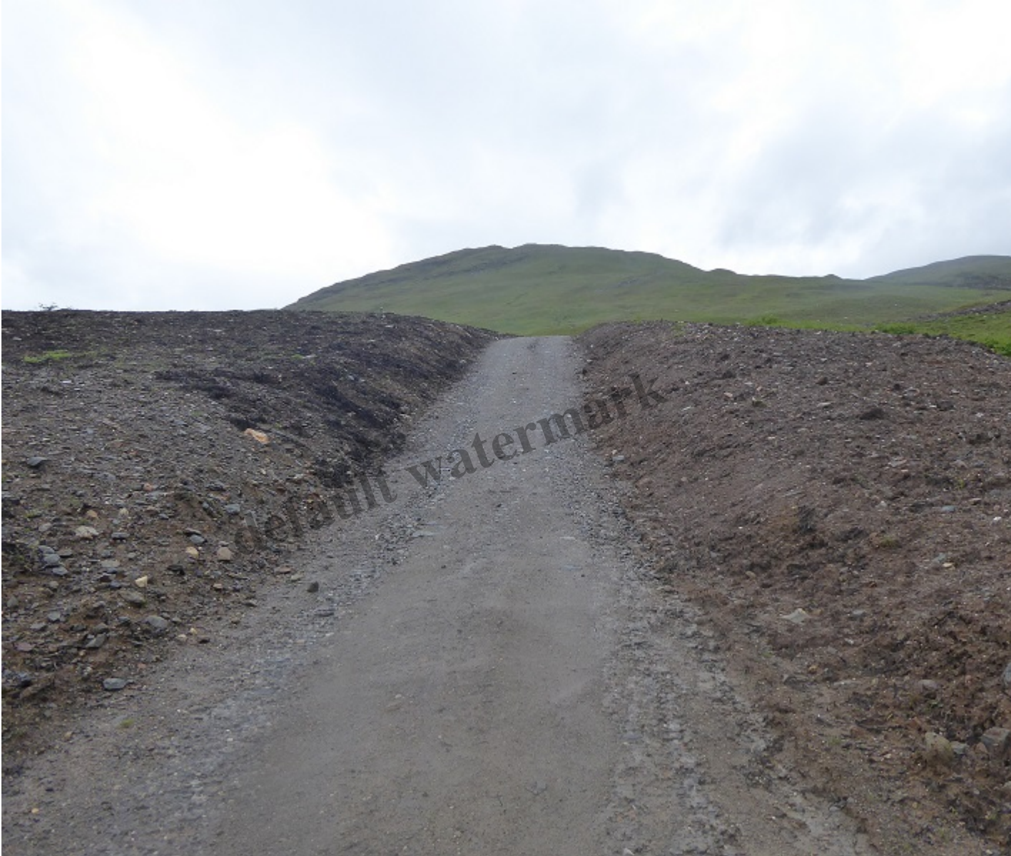
Bare ground all along the track results from the failure of the LLTNPA to enforce the planning condition that the turf be retained and stored properly.
