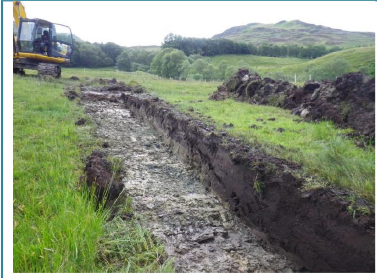
Photo from report of site visits in August 2015 at initial stage of construction
