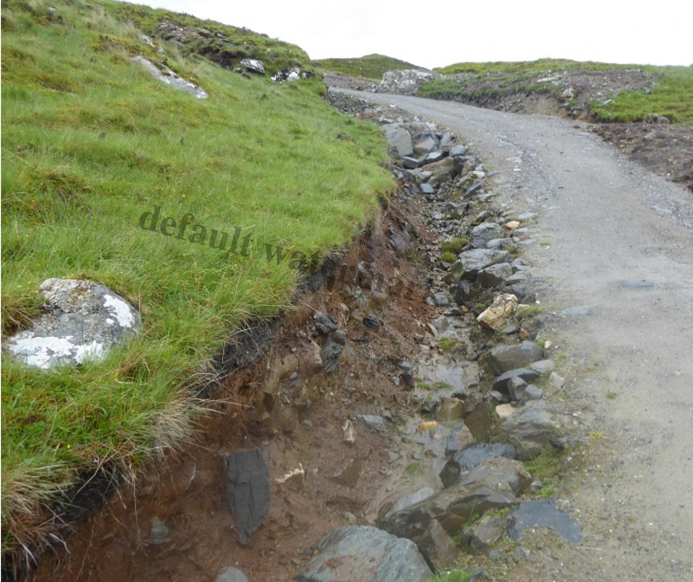
While this section of track has been narrowed the section of bank on the left is too steep, the edge of the track is crudely done and it's too steep – you can see how it was already washing out before it bends left.
