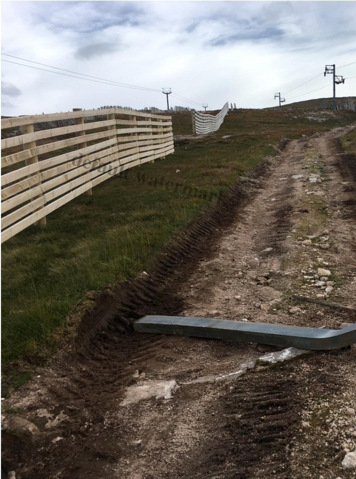
Damage to edges of existing track by vehicles which appear to be driving out the demolition material report (point 8) stated the materials would be airlifted out.
