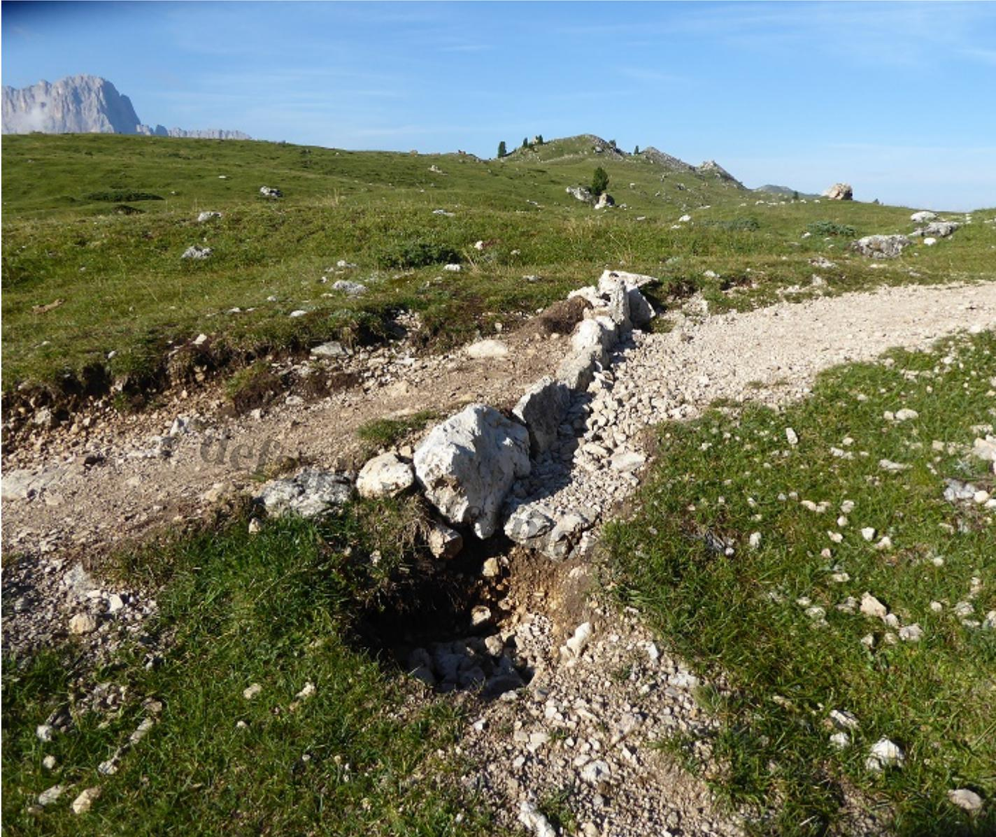
Evidence of recent maintenance work could be seen along many paths: here a drainage hole has been dug in order to create a sump for water running off a path
