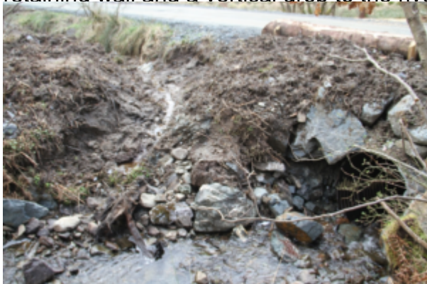
Attempts at restoring vegetation over this hardcore has been
