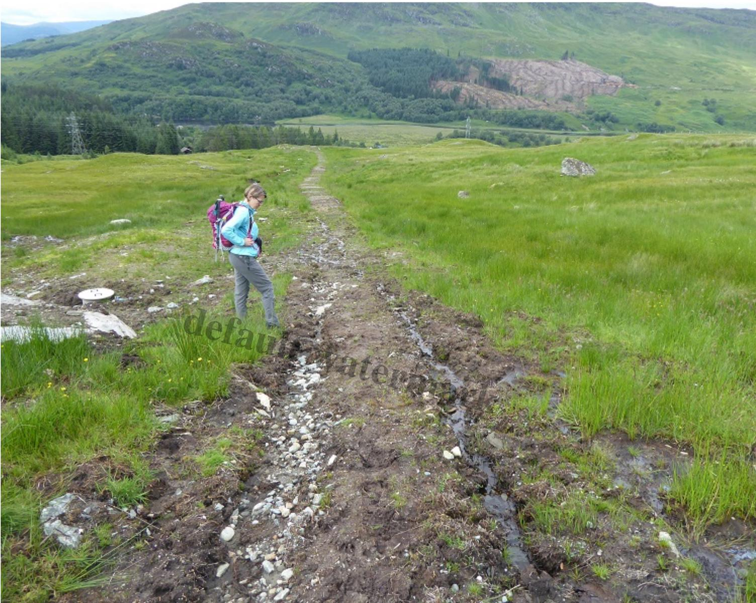
The recovery of the ground above the pipeline and construction track is not as good as it might have been because vehicles have been driven over land which is far too wet to support them.
