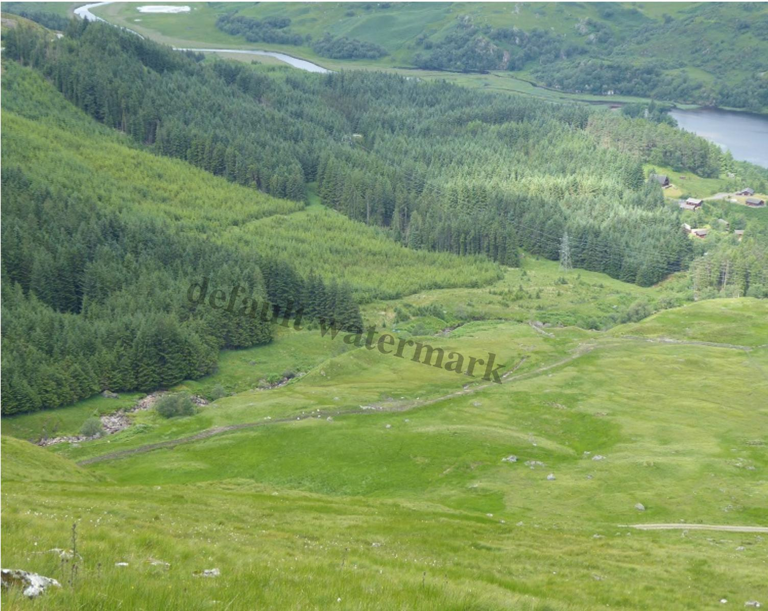
The construction track was along the line of the pipeline and was removed completely. The ground is recovering well. The existing hill track â?? bottom right â?? was not used for the construction although it runs round the hill not far from the intake.
