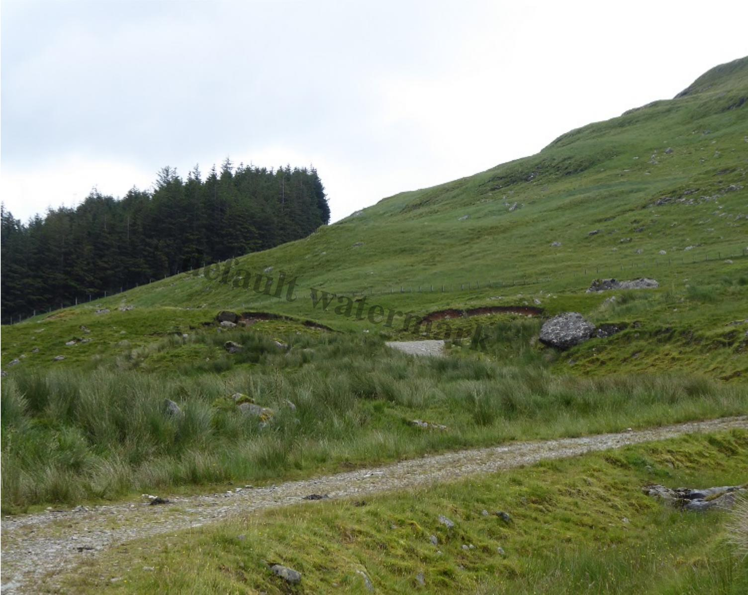
Having visited the site I have become more concerned. The construction track will cut across the hillside from just after the top of the last zigzag on the existing track to just above the top of the plantation. This is steep ground. It means cutting a great bench into the hillside. There are diagrams illustrating this in the application but no indication of how long each steep cross section will be:
