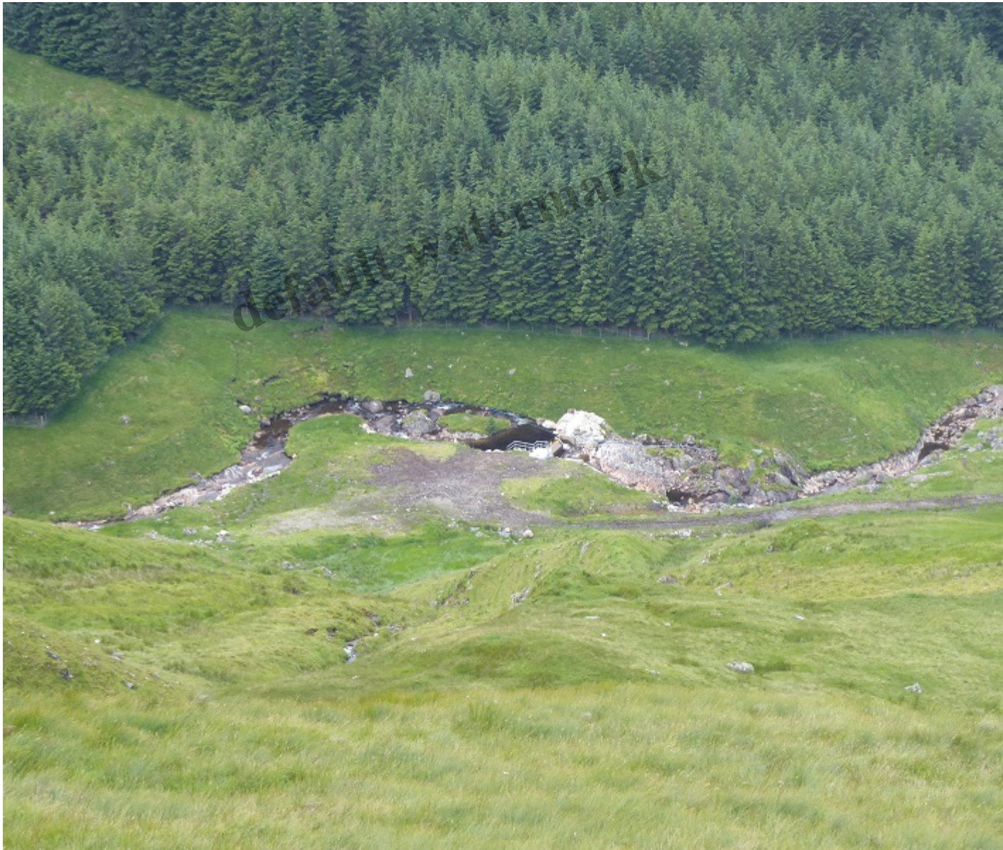
View of the intake from north west shoulder Ben More.
