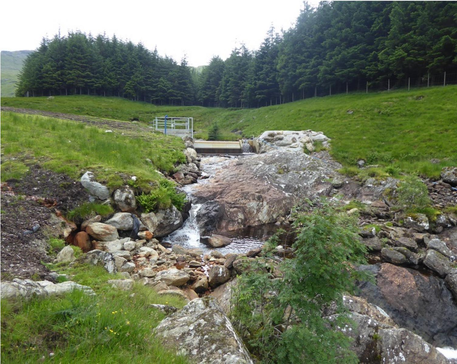
One thing I really liked about the intake was that instead of the normal concrete retaining wall, the development has embedded boulders in concrete. This creates a far more natural form. You can also see the browner rock below the intake which appears to mark the former "normal" flow levels of the burn. The hydro schemes are having a significant impact on river flows which will affect their ecology. I don't believe we really know yet what the permanent impacts might be.
