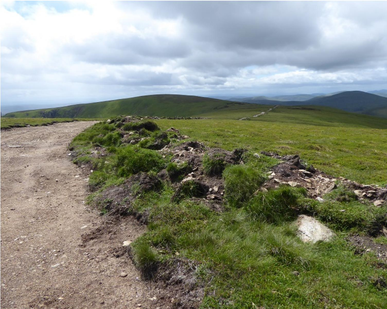
The track has been created by a digger scraping off the turf and dumping it by the side of the new track. The positive thing about this is it should make restoration of the track quite simple. All the estate would have to do is replace the turves and soil onto the bare surface.
