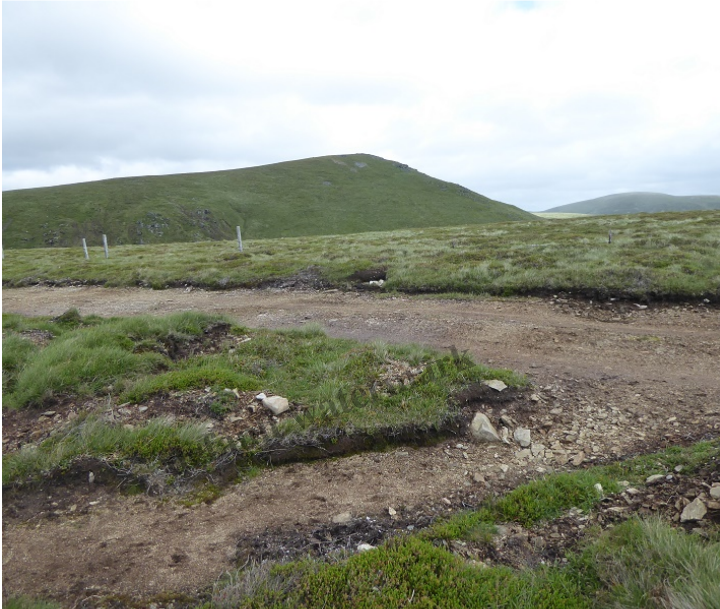
View across track to Mayar. The creation of drainage channels adds to the mess and impact on veg
