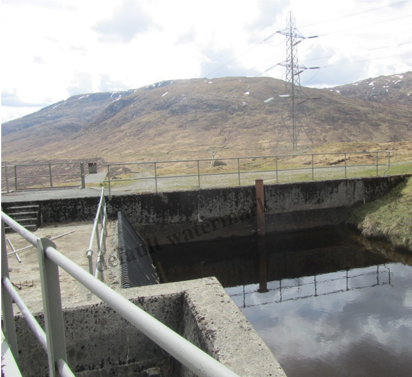
Alt nan Caoran Hydro intake south of Ben Lui and Ben Oss – you can just see pipeline above centre
