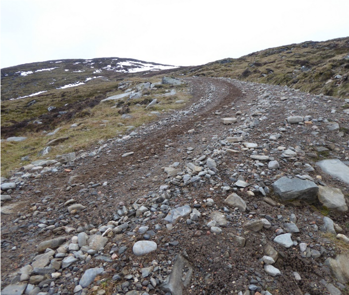
The lower section of the track up the shoulder of Craig Leth Choin is apart from the landscape impact and will be constantly subject to erosion
