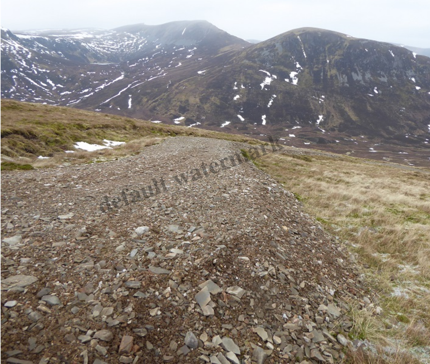
Part of upper section of Cluny Estate track, Glen Banchor
