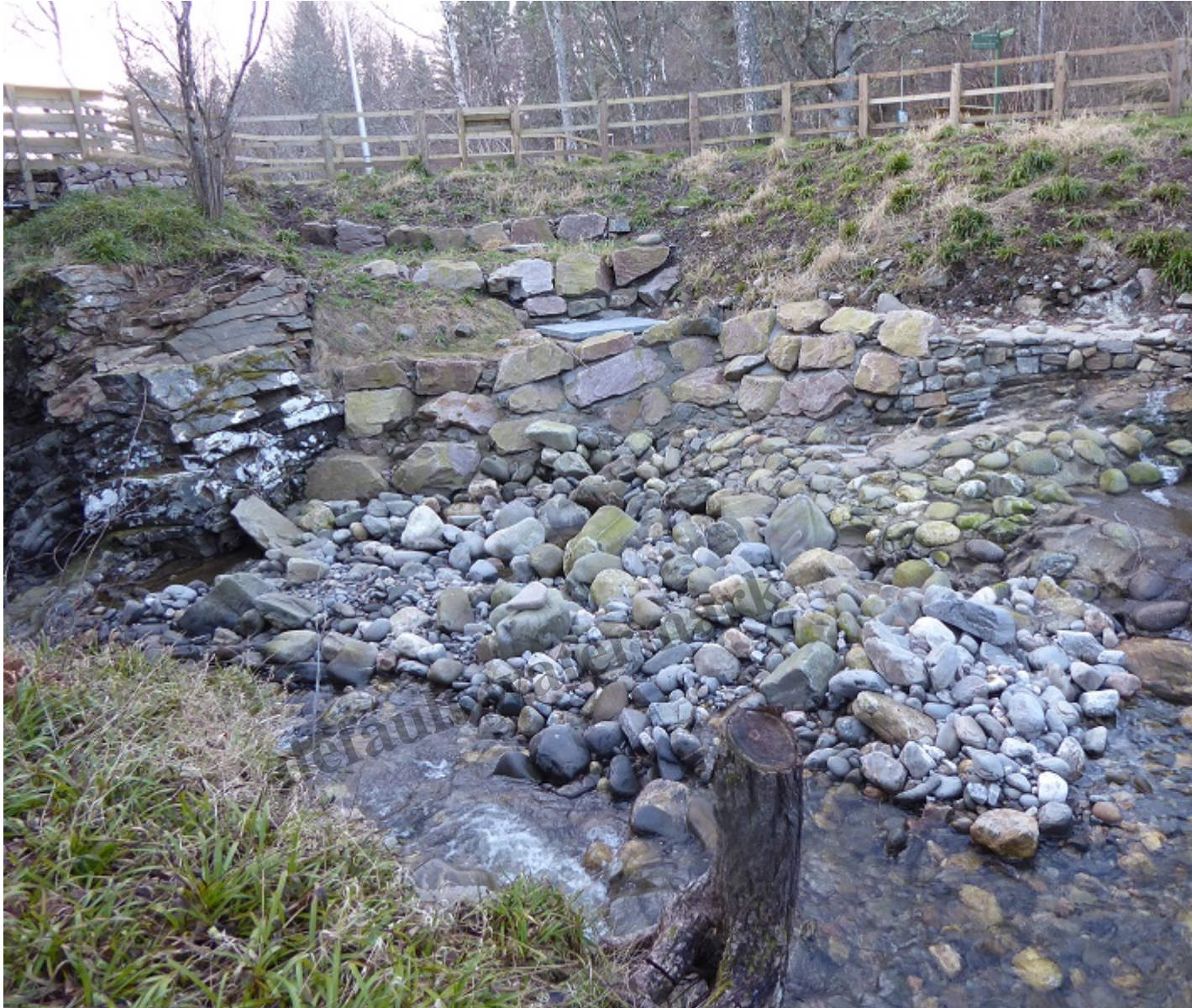
The line of the pipe, viewed from close to the intake, runs behind the line of the wall on the right.
