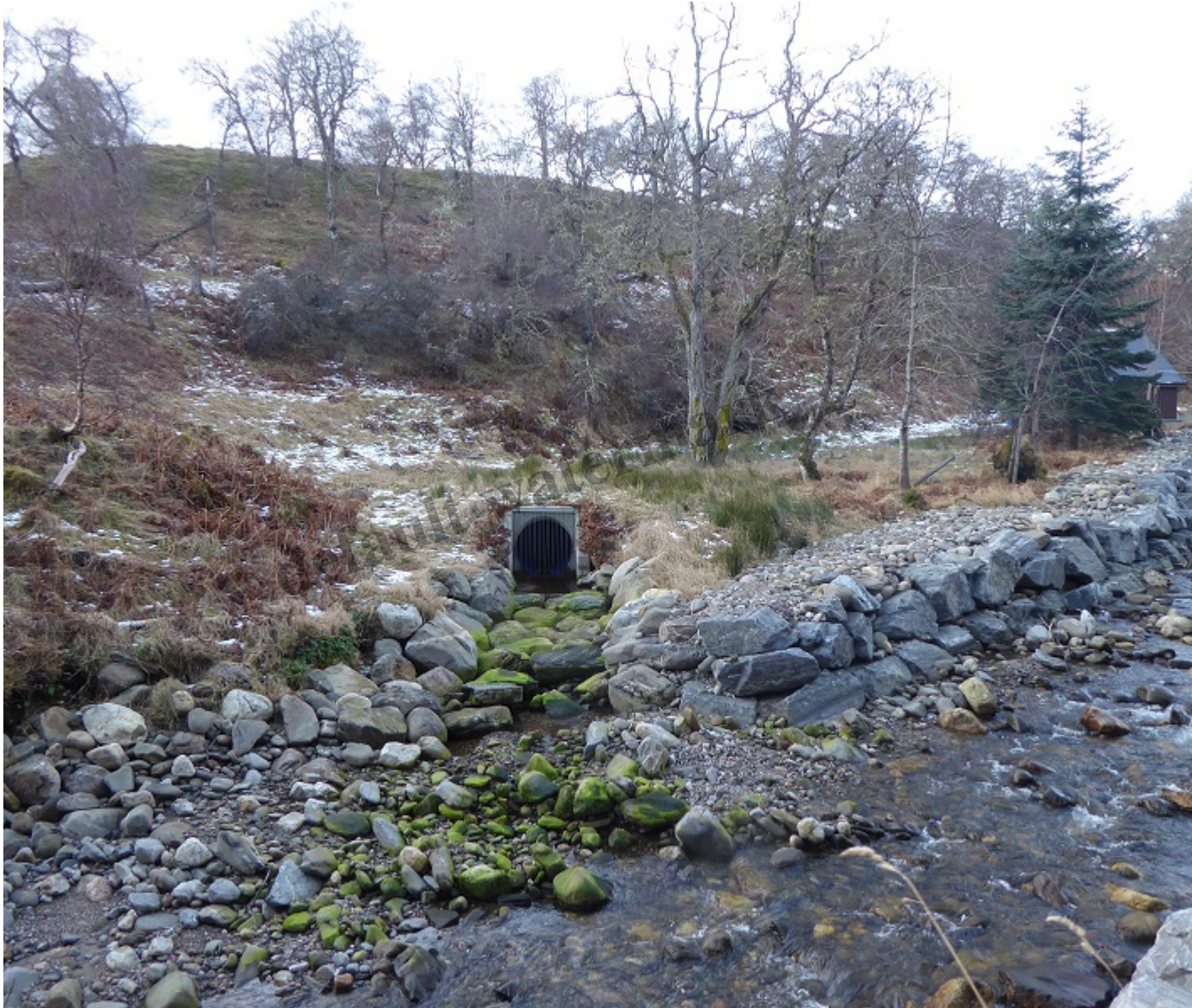
View from east side River Gynack of tailrace and powerhouse. The rip rap bouldering along the river is the hydro scheme.
