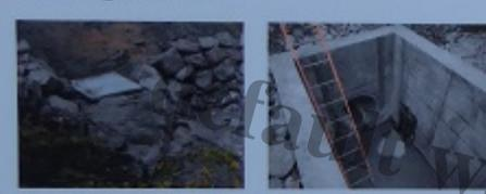
The purpose of the settling chamber, which has a volume of 10000 litres, is to remove turbulence and air that arises from the flow through the Coanda screen, thus allowing water to flow smoothly down to the turbine. It also allows any sediment that settles out to be collected and flushed out a side pipe back into the river. The water level in the chamber is controlled at a constant level by operation of the turbine vanes.
