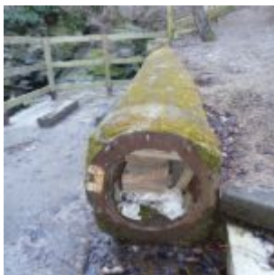
The section of former pipe
