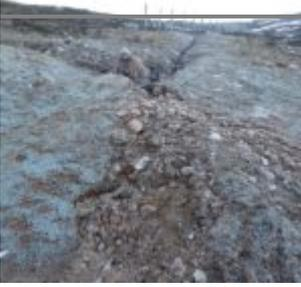
Water overflowing the drain created above the bulldozed slope and running down
