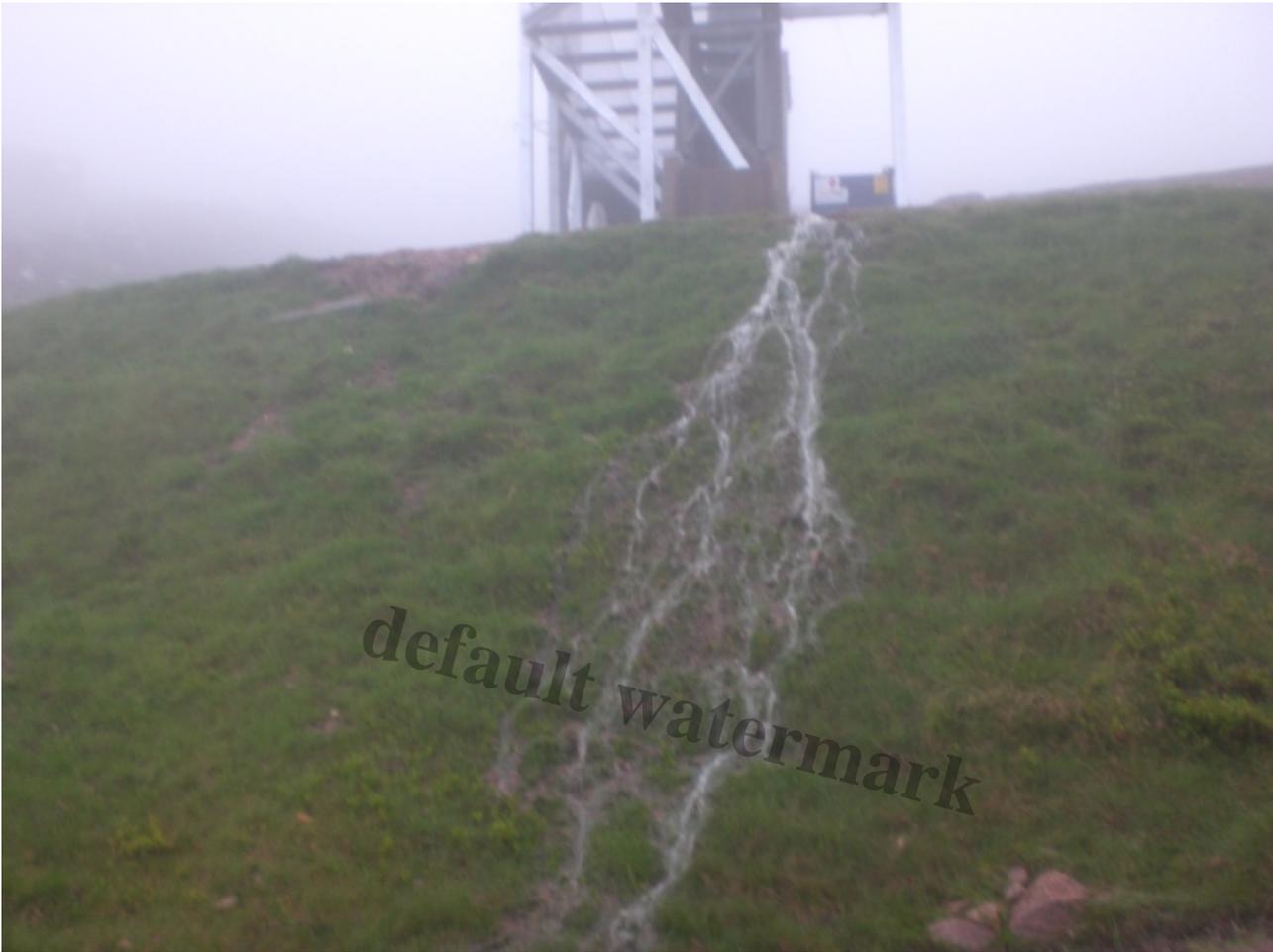
Below the gantry, the water runs down the bank which was re-seeded at an earlier date. This has helped limit the damage but for how long? No slope as steep as this will be able to withstand this amount of water for long. The problem is the works at Cairngorm, channelling water onto new ground which will not be able to withstand its erosive force.
