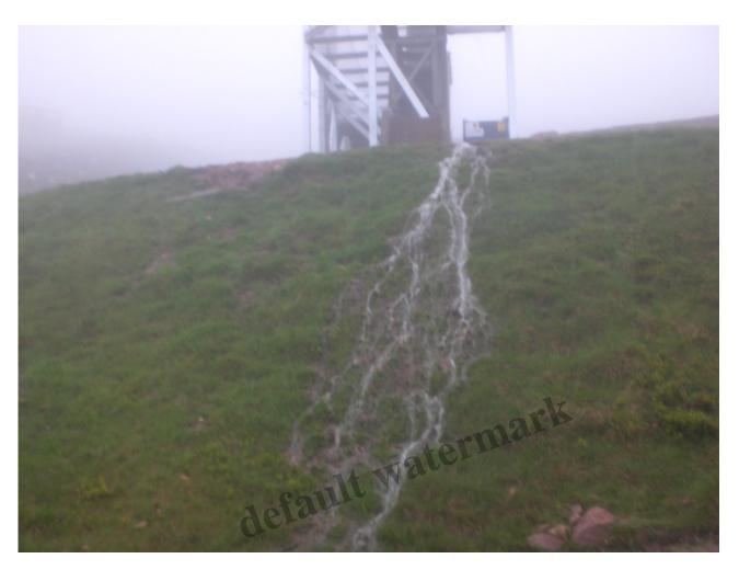
Below the gantry, the water runs down the bank which was re-seeded at an earlier date. This has helped limit the damage but for how long? No slope as steep as this will be able to withstand this amount of water for long. The problem is the works at Cairngorm have altered the pattern of water flows at Cairngorm, channelling water onto new ground which will not be able to withstand its erosive force.
