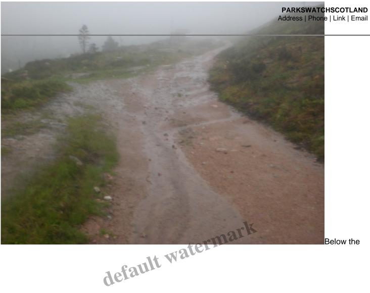
bottom of the Shieling rope tow (far distance) and by the unlawfully re-graded bank, the track has become a burn. You can see how water from the bank which Natural Retreats claimed they had "improved" is flowing onto the track. There is no way of measuring how this compares to what happened before, but the destruction of vegetation on the bank is likely to have increased the rate of water run-off.
