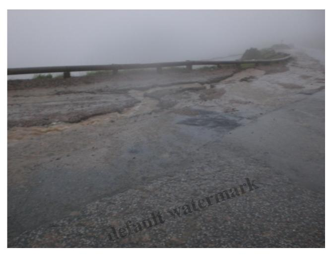
All this increased water run off is not only increasing erosion of the natural environment, its impacting on humans. The bottom of the Cas carpark was a raging torrent and is.being washed away and down into the lower Cas carpark. Below that of course is the Allt Coire Cas and the people of Aviemore.
