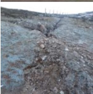
Water overflowing the drain created above the bulldozed slope and running down
