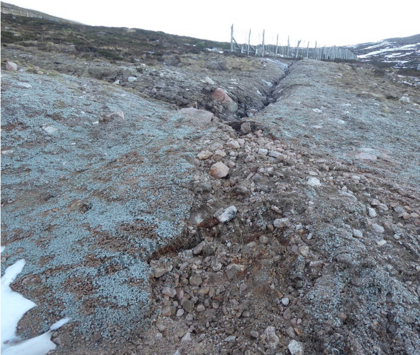
Erosion on the slope to the right of the Cas Gantry January 2017, with blue fertiliser pellets washed a
