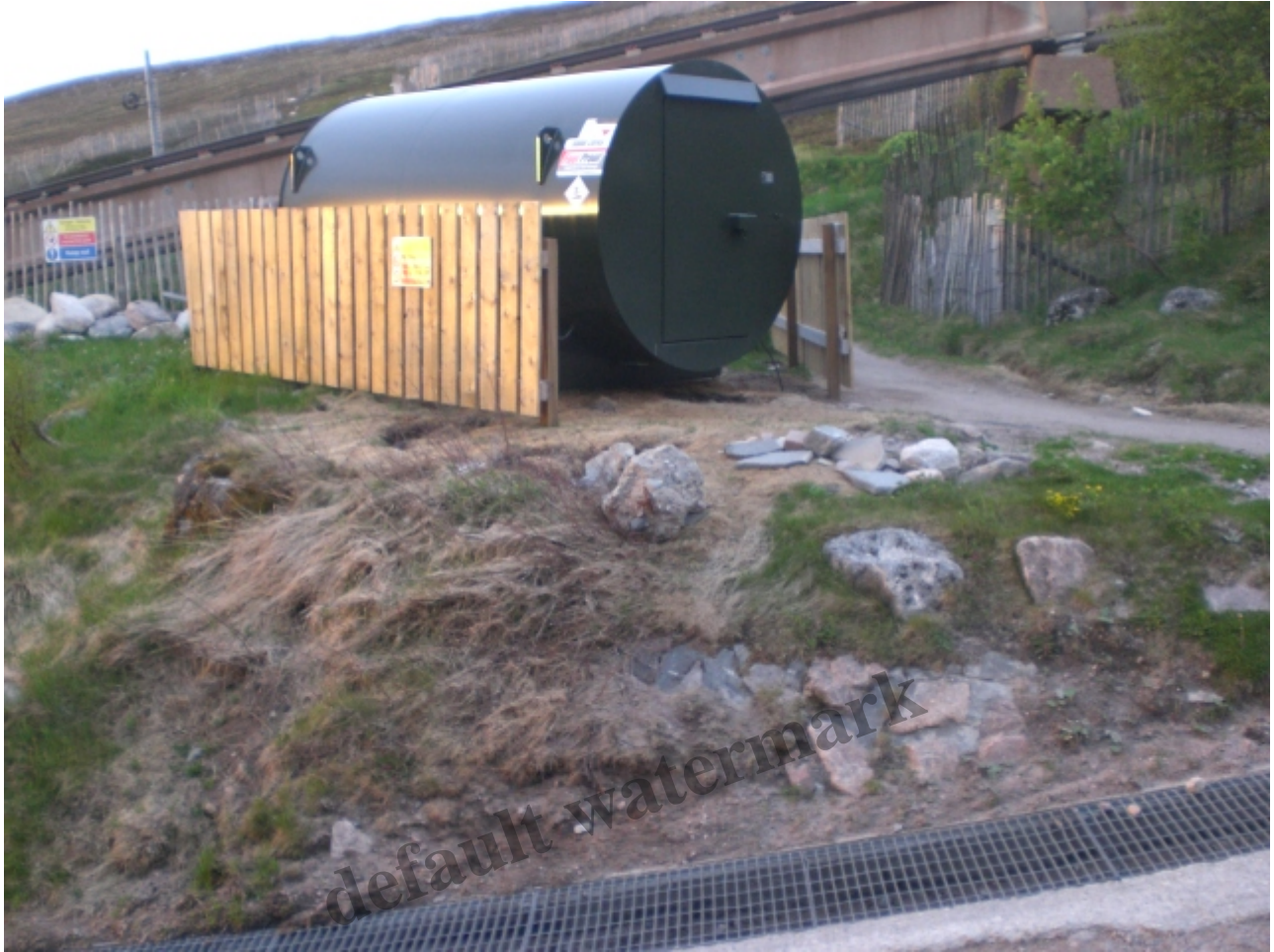
Diesel tank adjacent to funicular station – note dead vegetation centre and left
