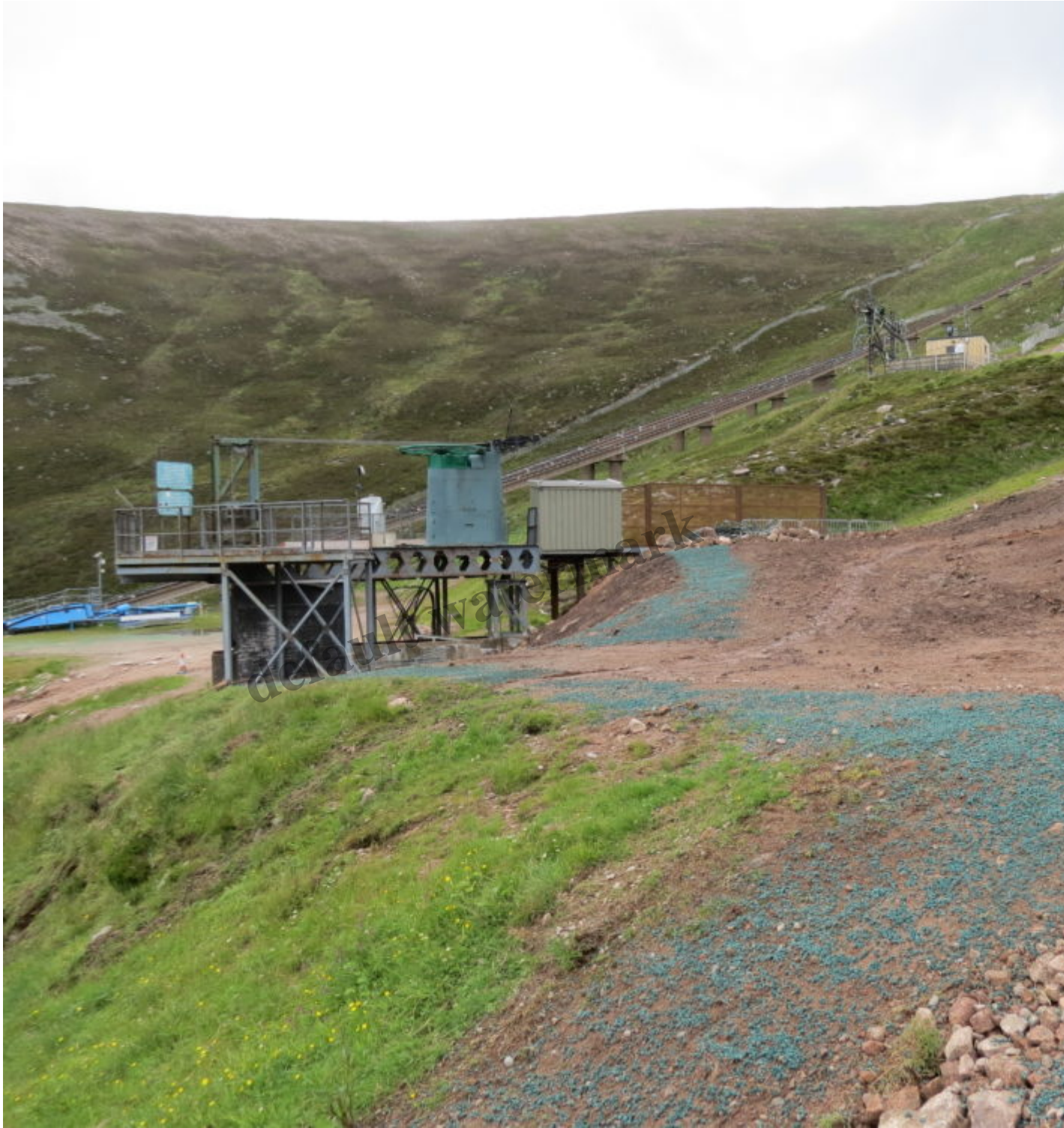
View of Cas Gantry August 2016
