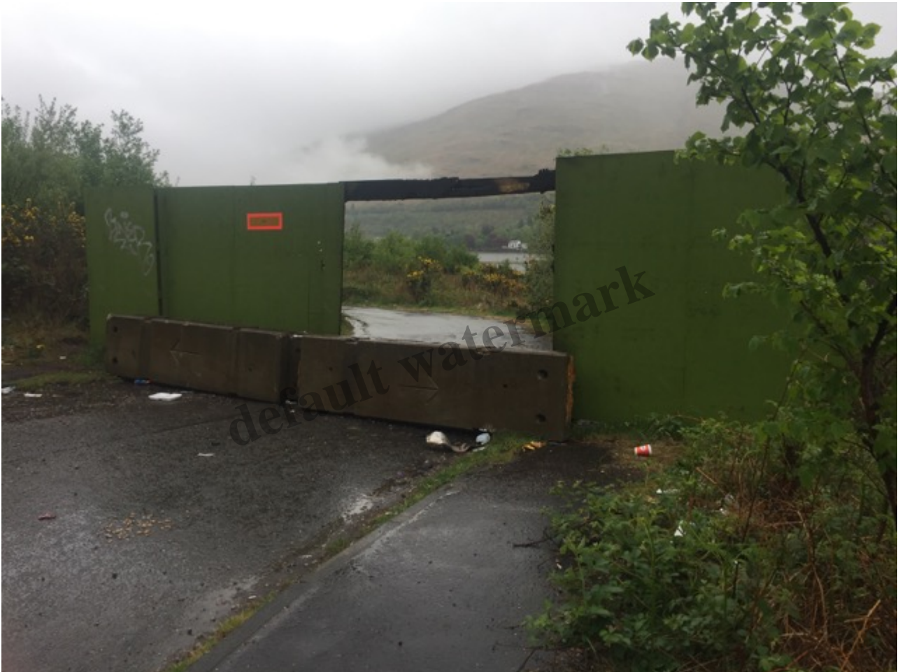
Southern entrance to torpedo station site 15th May
