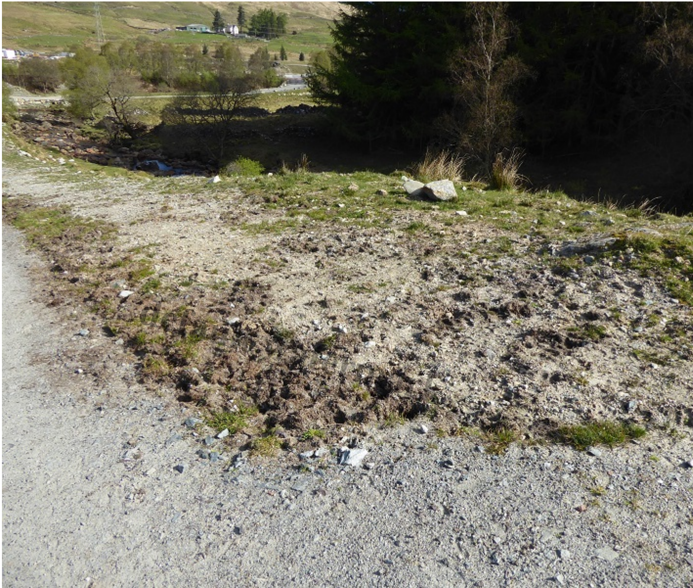
Photo showing how original attempt to cover former track surface is failing, with former surface of co track being revealed as turf has been eroded by cattle.
