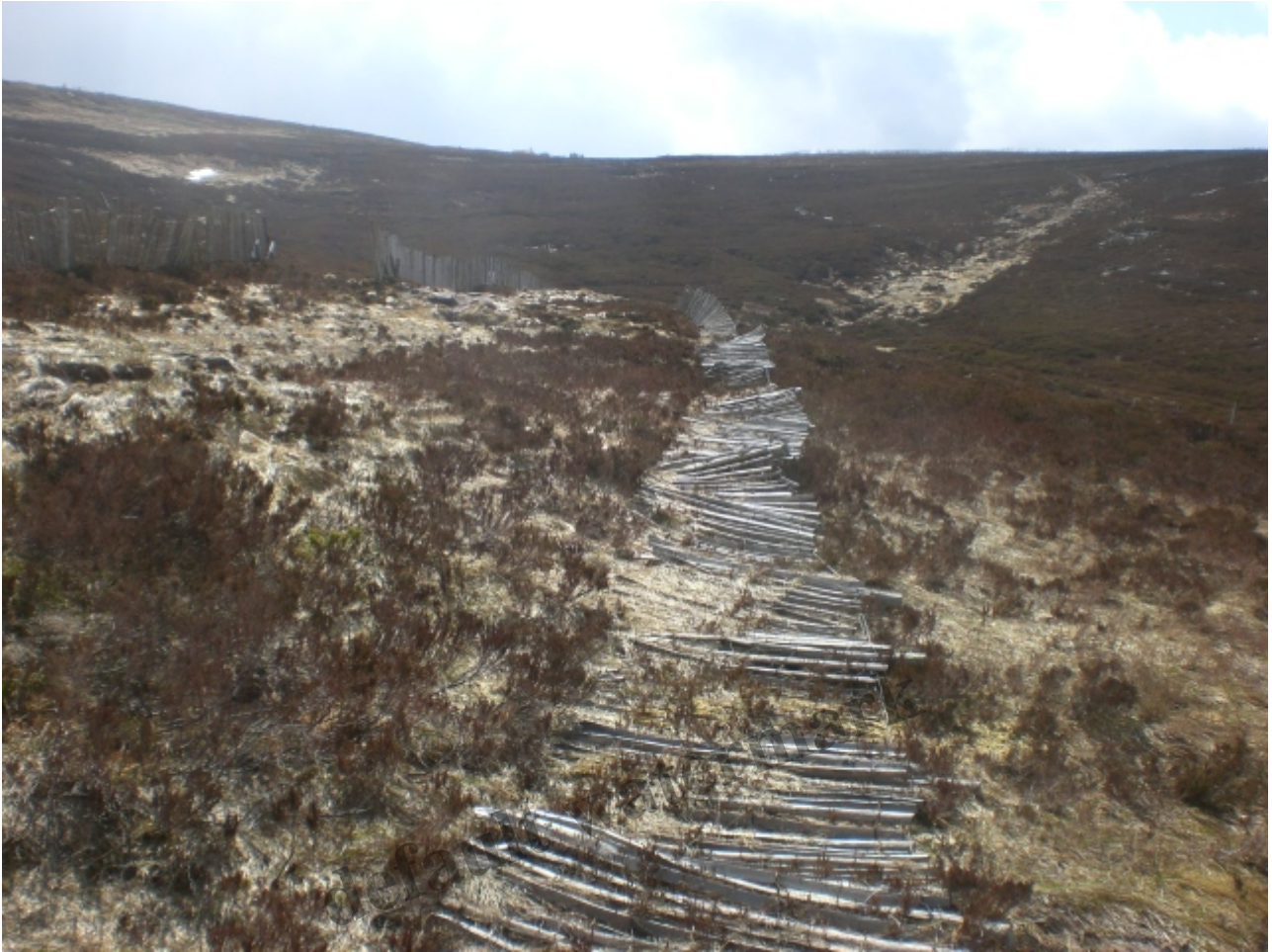
Collapsed snow fencing, approaching West Wall poma upload area
