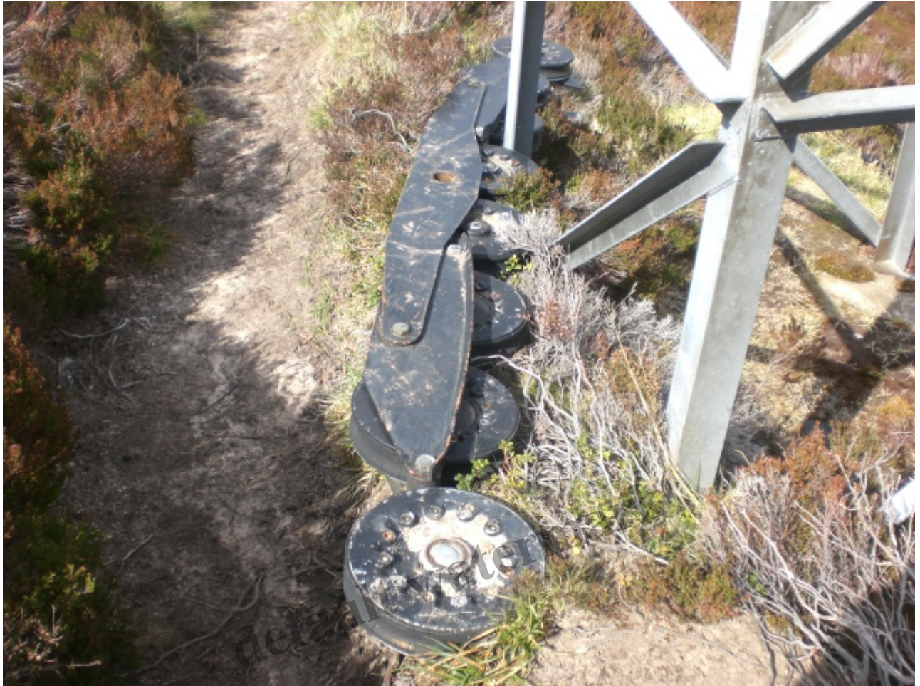
Abandoned chairlift sheaves which have been on the ground since 2012
