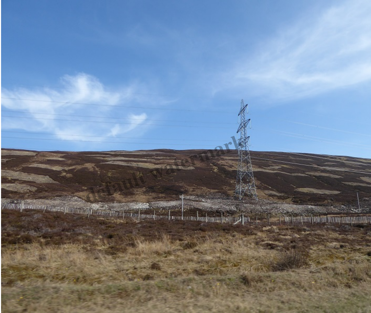
Travelling down the A9 on 1st May I took photos of almost every tower you can see from the road. The condition of soils and vegetation is not hard to see as with this pylon south of North Drumochter Lodge
