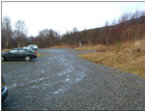
Existing Car Park
