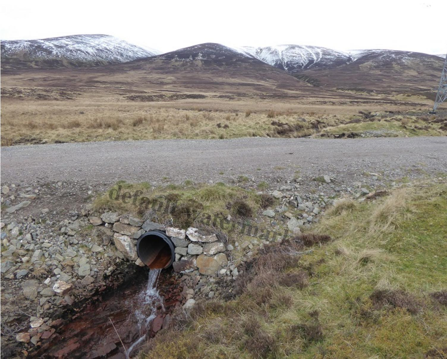
Bizarrely, among all the protruding pipes, there was one example of a culvert which had been properly finished – at both ends too! Unfortunately, the track here was even wider than normal, 7m rather than 5m, and at least one of the finished culverts will need be ripped out if the track is to be reduced in width to 3m. If this work was done by SSE, one wonders why? If by the Estate, that would suggest they are intending to keep the track at its current width, contrary to planning requirements.
