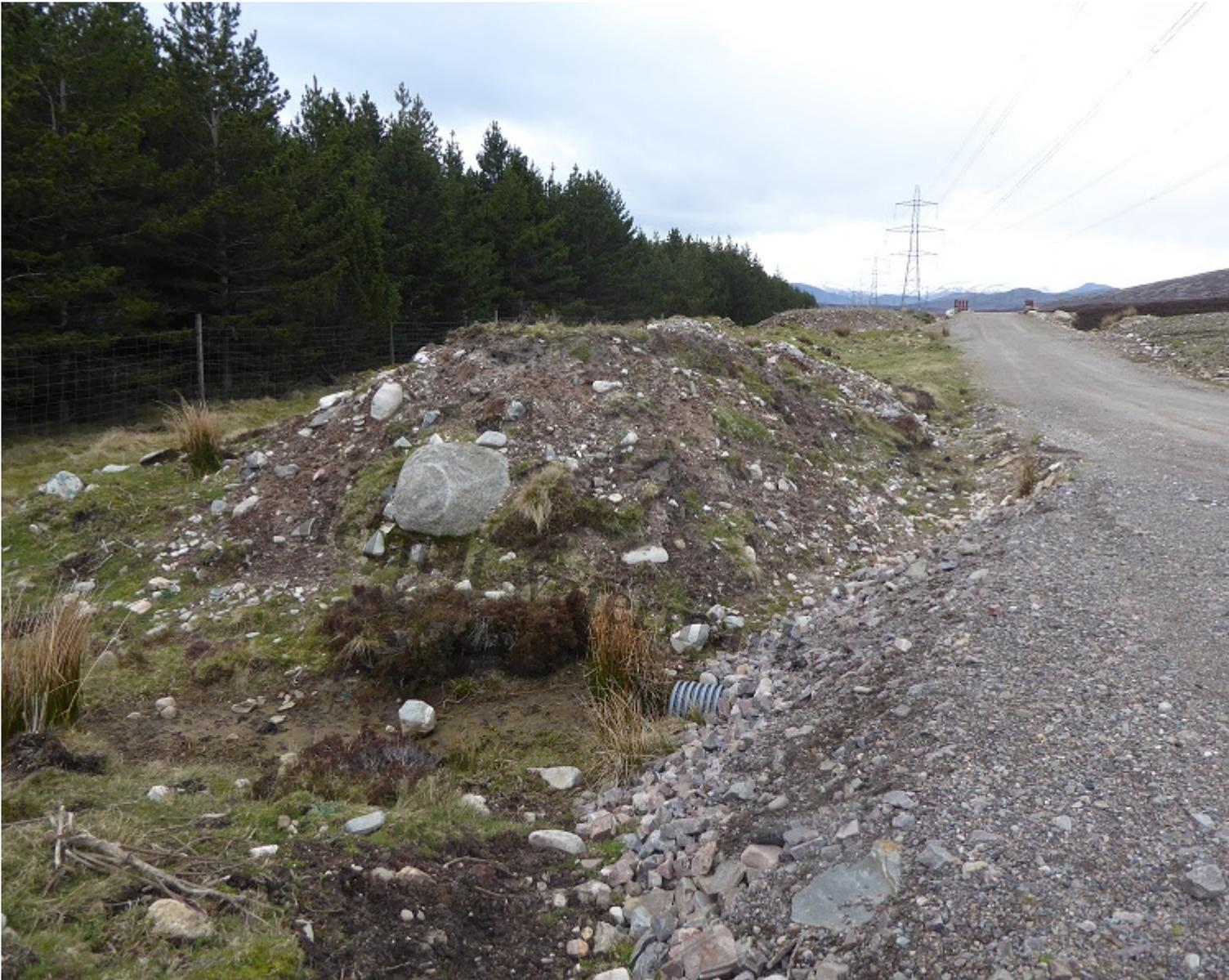
The amount of work â?? and therefore cost â?? in meeting the approved design plans for the track are considerable. The 4.7 km of track needs to be reduced from its current width of 5-7m to 3m.
