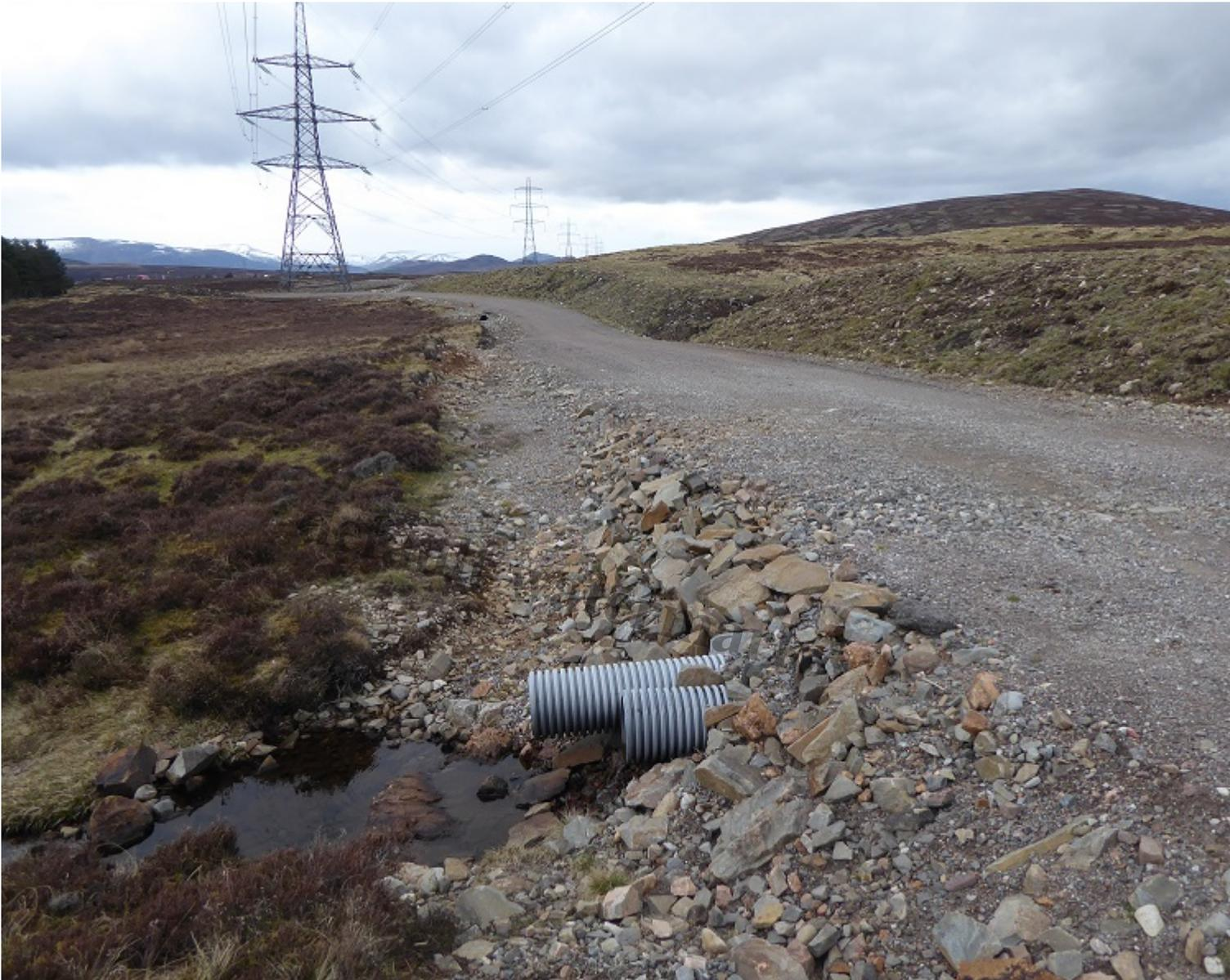
The job will not be made any easier because so much of the temporary construction work was so poor. If this track is to be halved in width, so will the drainage pipes.
