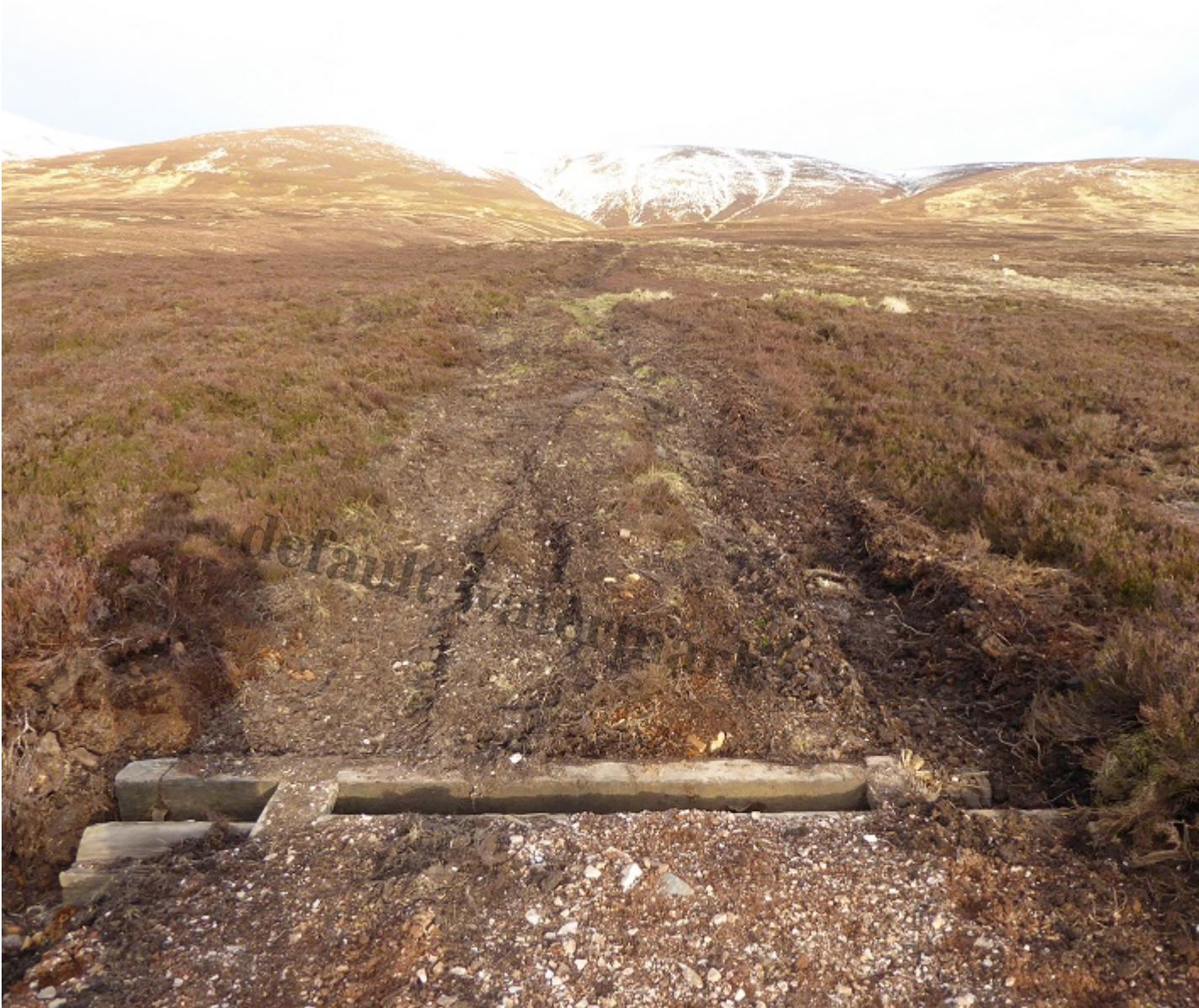
End of the 20m section of track showing erosion created beyond
