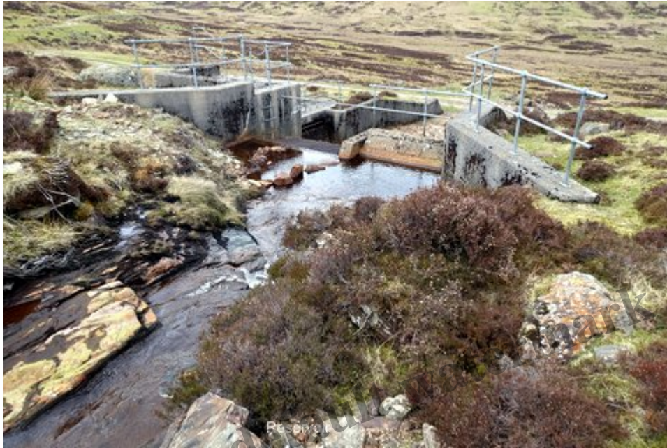
View from above intake – Photo Credit Jim Robertson
