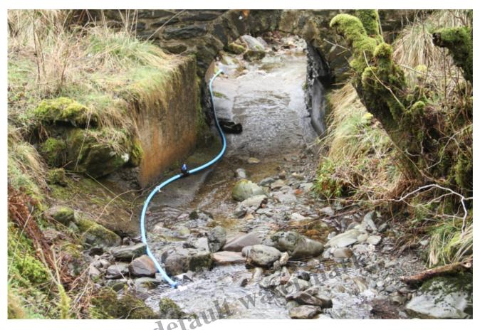
An unsightly installation with loops in blue water pipe makes a poor impression. When taken together with the positioning of the intake manifold, which is partially out of the water, unsecured and likely to be dislodged the first time the stream is in spate, it provides a rather damming but realistic indication of what was initially installed.
