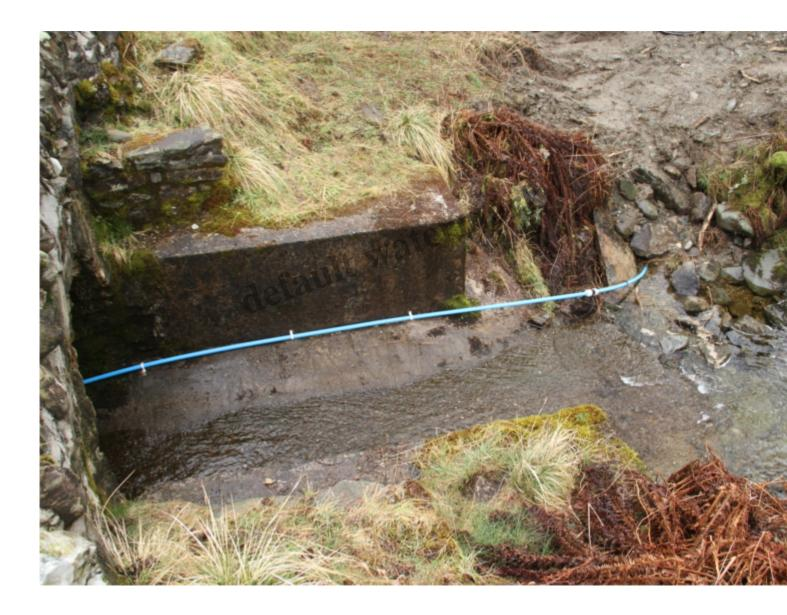
Of course once the air lock is in the system it won't self clear easily as water won't flow up hill. So many basic principles have just been overlooked cumulatively resulting in poor system design. This is a contributory factor together with the failure of staff, the clerk of works and the contractor to understand the basic requirements for implementing such a water supply.
