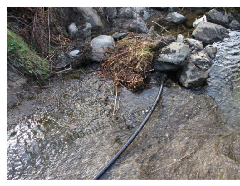
The arrangement of the pipe has changed, now entering the river bank at a much lower level, the pipe is not secured on it's traverse across the culvert and the gap underneath will most likely collect sticks and other vegetation then a build up of debris will possibly occur.
