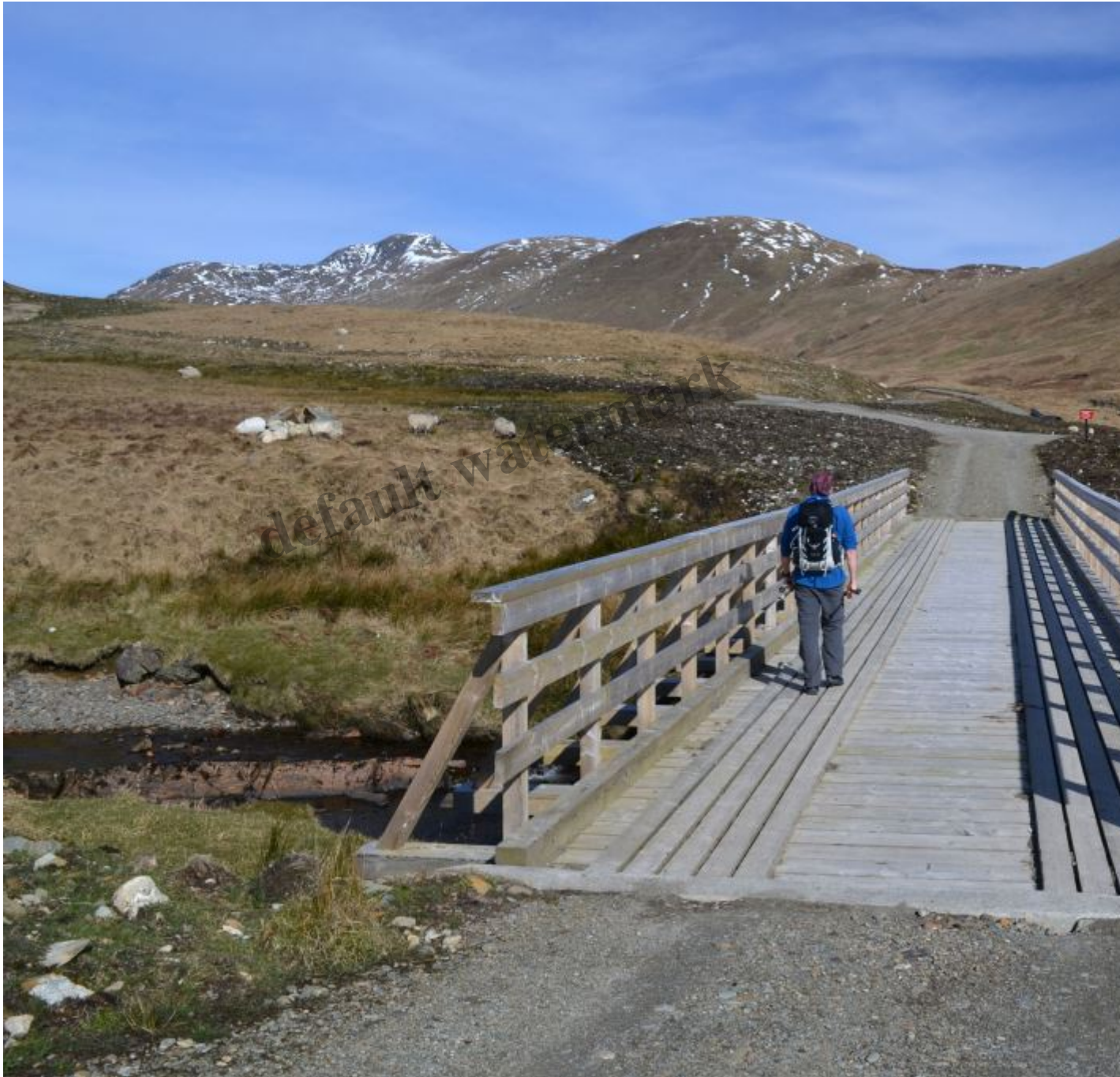
New bridge over the Allt Breac Nic, Stuc a Chroin in distance. The pipe has been concealed under guidance. Photo Credit Derek Sime.
