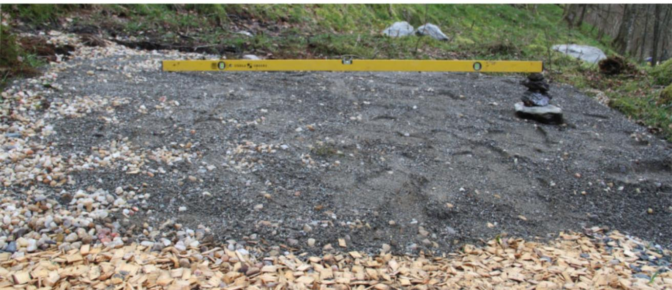
The problem with Pitch 14, as with so many at Loch Chon, is size and the slope. It's just too steep to be a viable camping pitch. In an attempt to make the pitch surface even, the Park Authority have covered the area with their inappropriate quartz aggregate / gravel mix and while it is now even they
