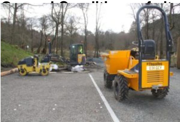
The area remains a building site with tracked vehicles,
