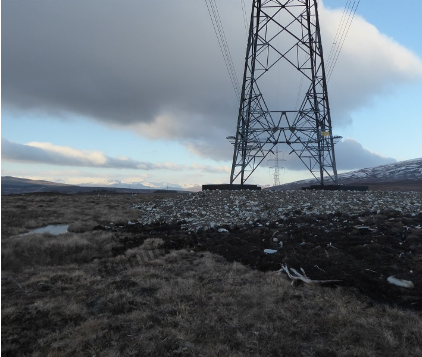
One of few examples at Drumochter where there is evidence of soils (in this case, peat, right foreground) restored although the restoration is only partial
