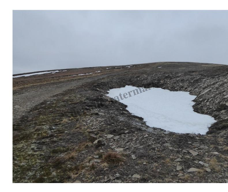
Taking what the CNPA has said at face value, there are serious challenges with restoring this track. The material that forms the track needs to be returned to the "borrow pits" from which it was sourced.
